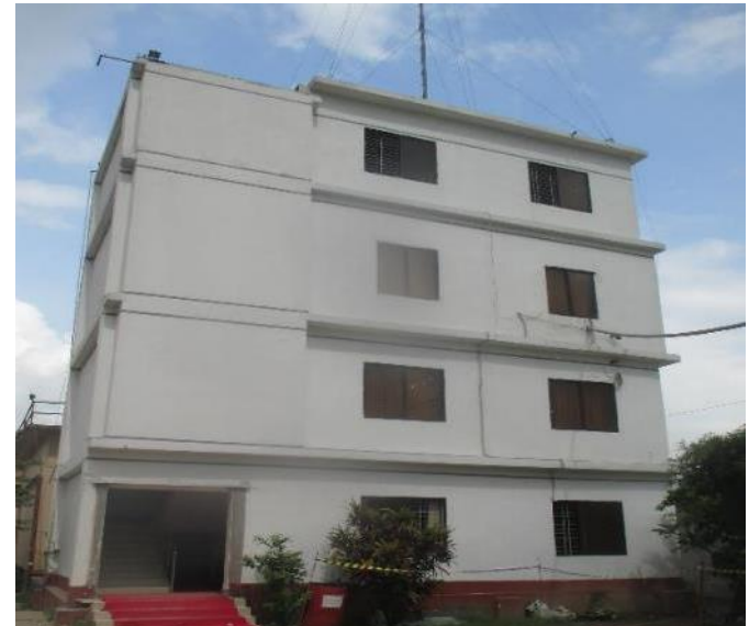
Office building was found as 4 storied
