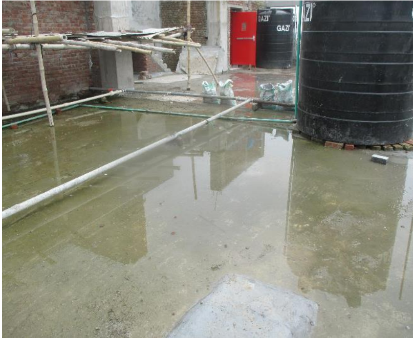
Water ponding on roof slab.
