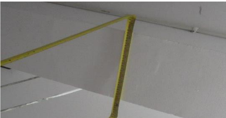
Width of NB was measured as 250 mm
