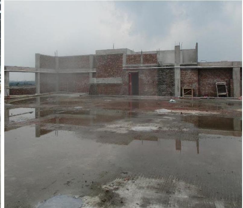
Water ponding on roof slab.
