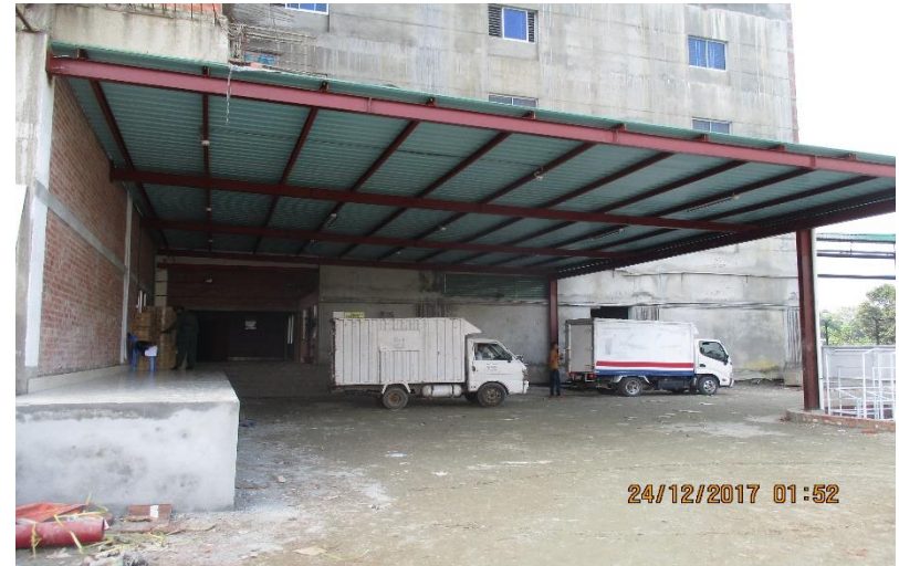
Canopy adjacent to main building
