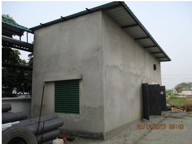
Boiler & compressor room
