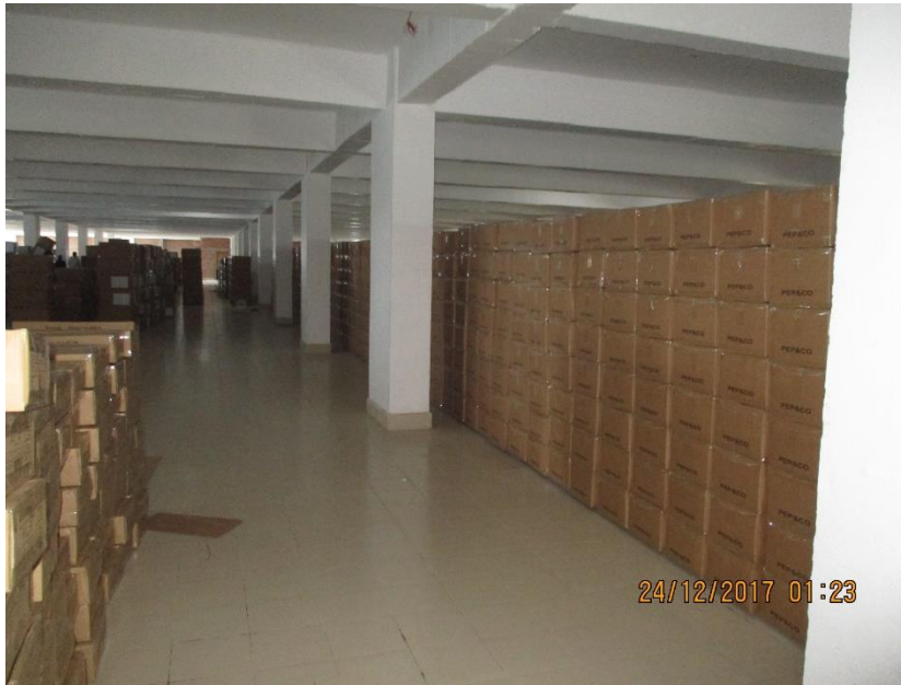
Uncontrolled live loading
