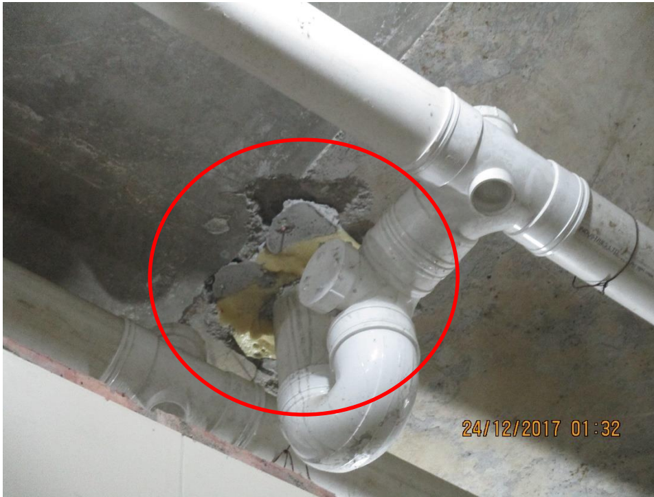
Concreting repair work
