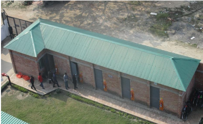
Wastage go-down & security room
