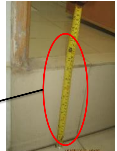
200mm built-up and 125mm thick outer brick wall on toilet area
