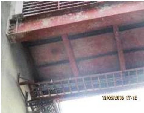
Connection of link bridge (at ware house portion)
