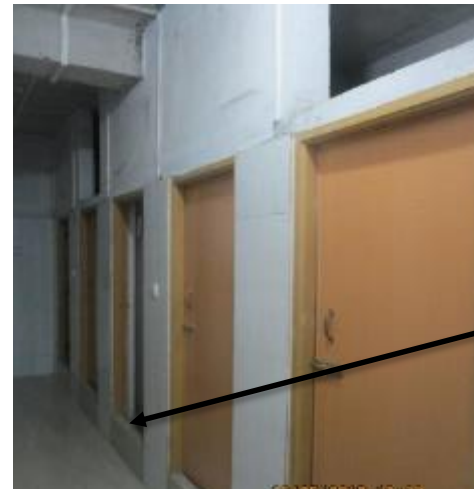
200mm built-up and 125mm thick outer brick wall on toilet area
