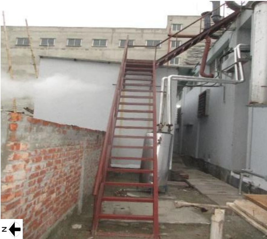
Steel stair beside generator room and canteen shed
