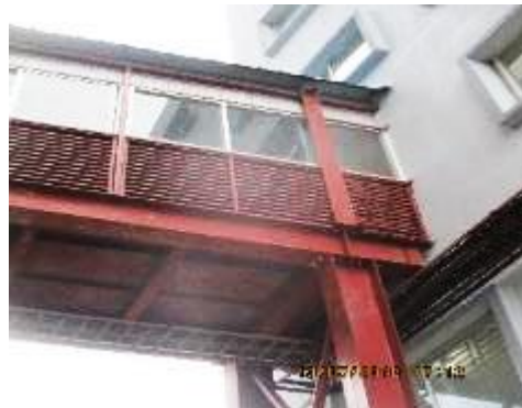
Connection of link bridge (production portion)
