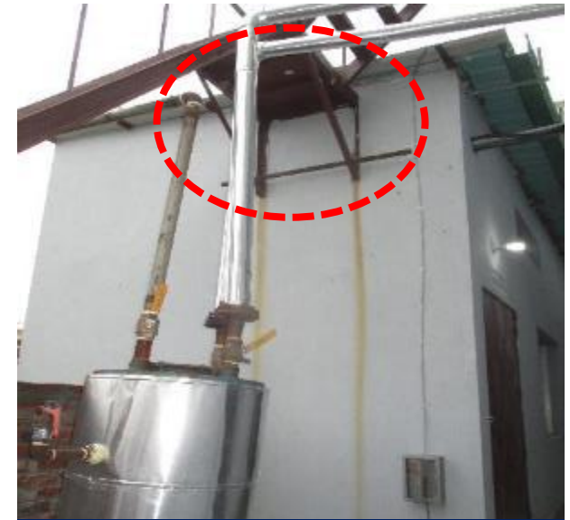
Bolted connection observed with brick wall to support the stair.
