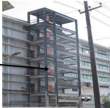
North-West side steel stair
