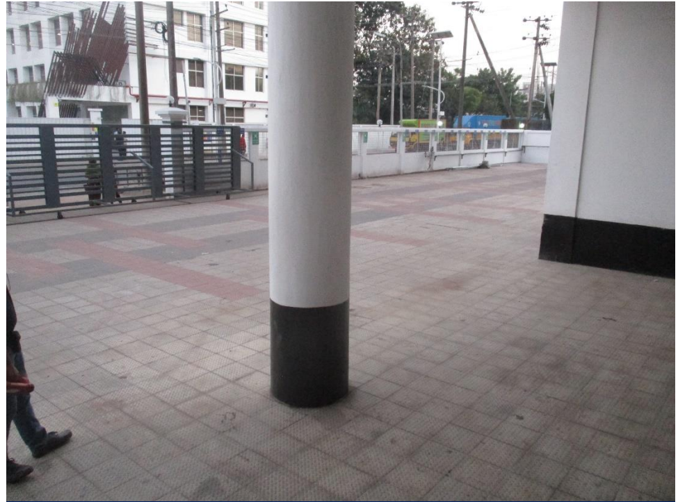
Ground floor column in loading-unloading bay.
