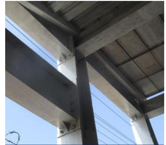
Bolted connection between column and beams.
