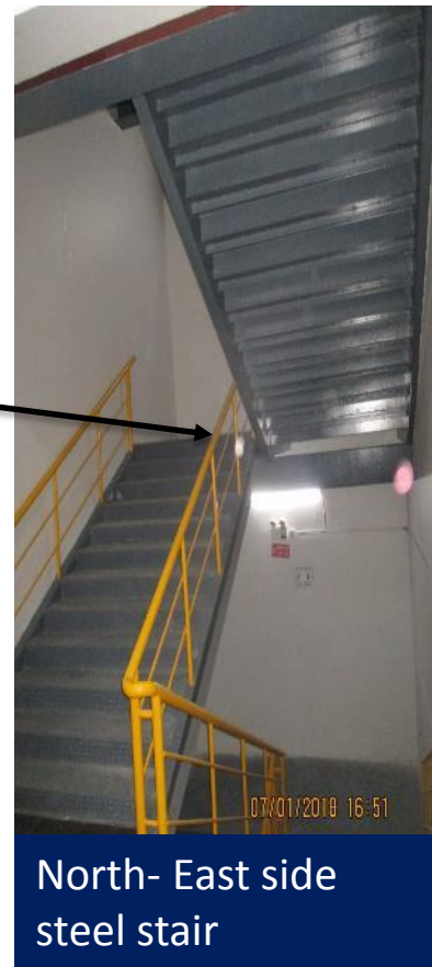
Steel column of the stair was installed adjacent with the RC column
