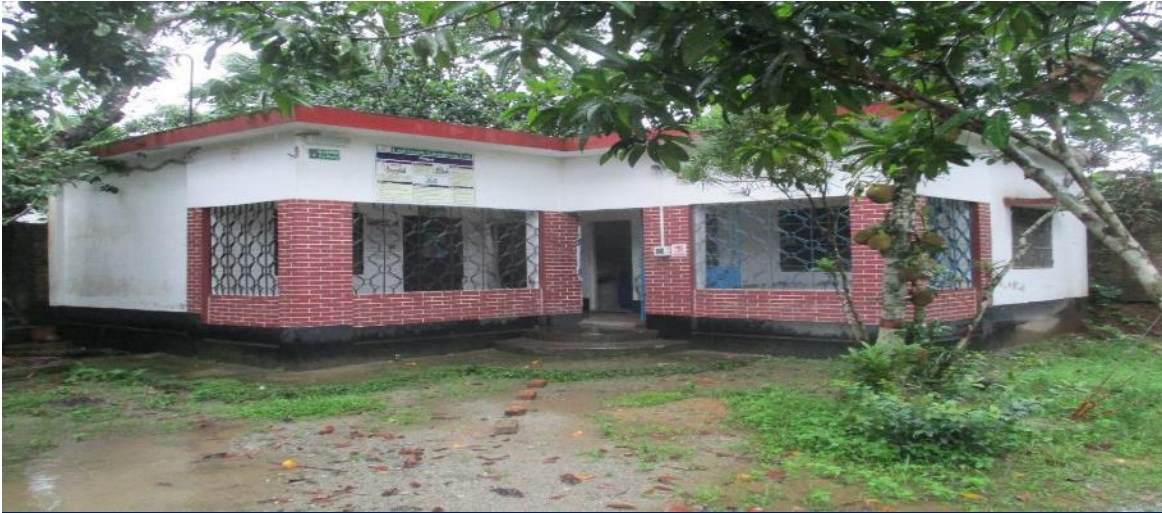
Extent of Childcare building
