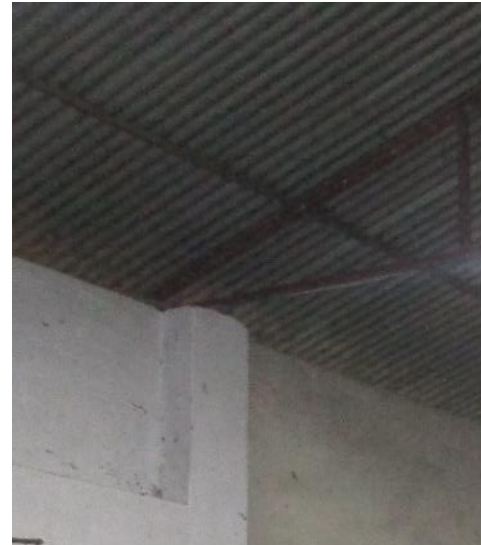
Roof truss supported by brick wall
