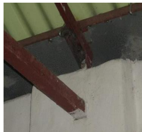
Truss supported on brick wall.
