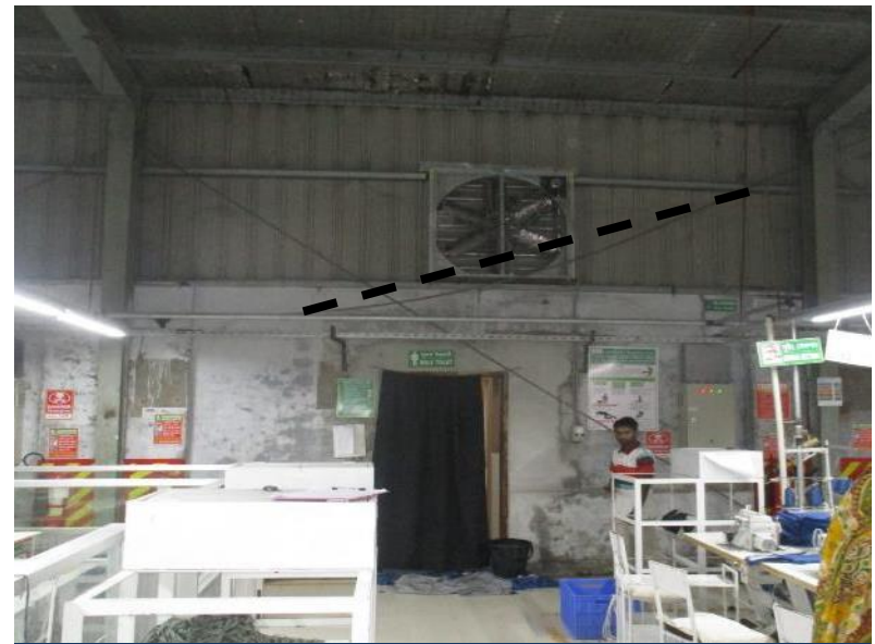
Discontinued Vertical bracing.
