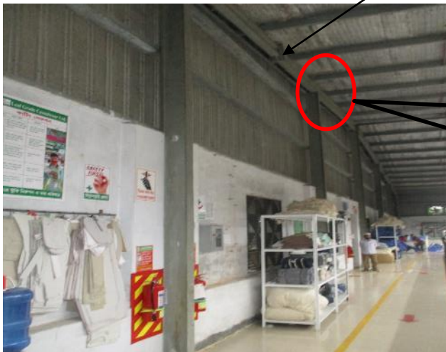
End wall framing at grid 1-1
