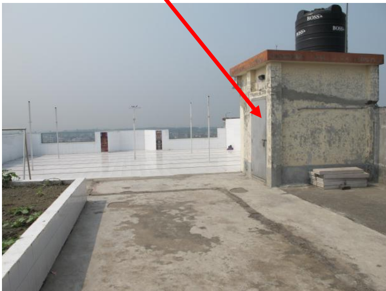
Store room and water tank
