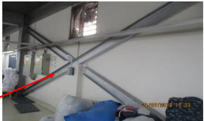
Vertical bracing on north side
