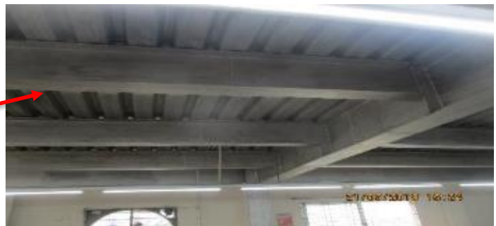
Deck slab system on steel part
