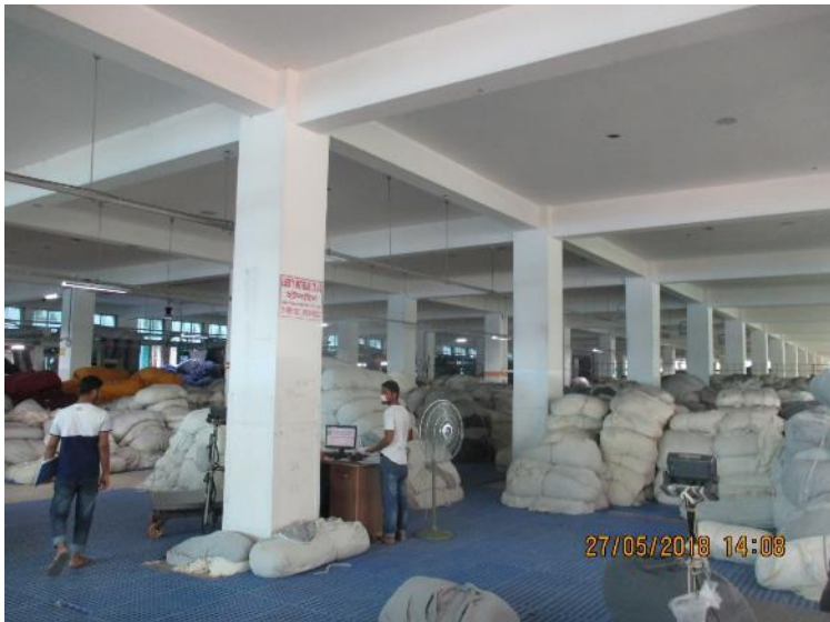
Typical beam-column framing system
