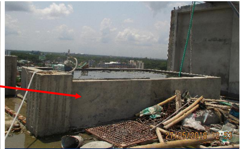
Temporary Water Tank
