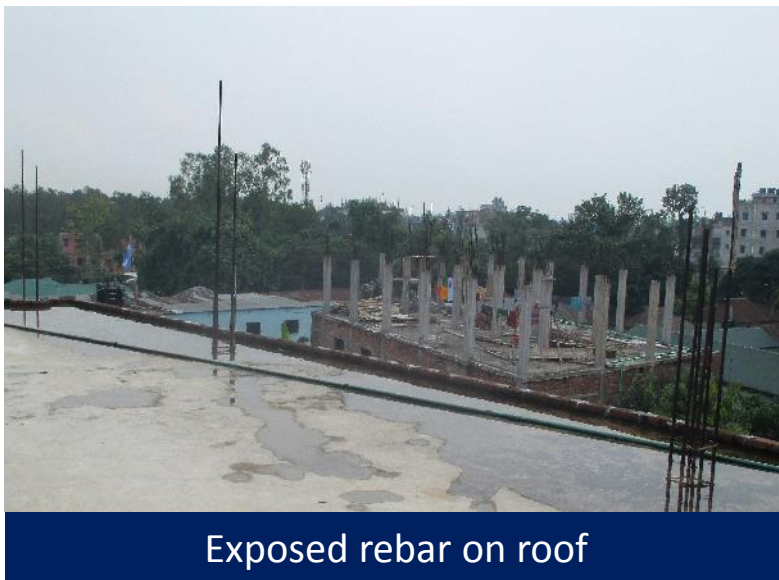
Water clogging on roof top
