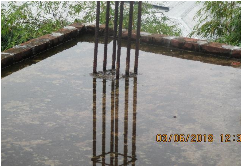
Water clogging on roof top
