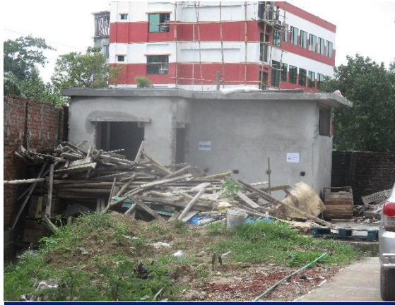
Fire pump room
