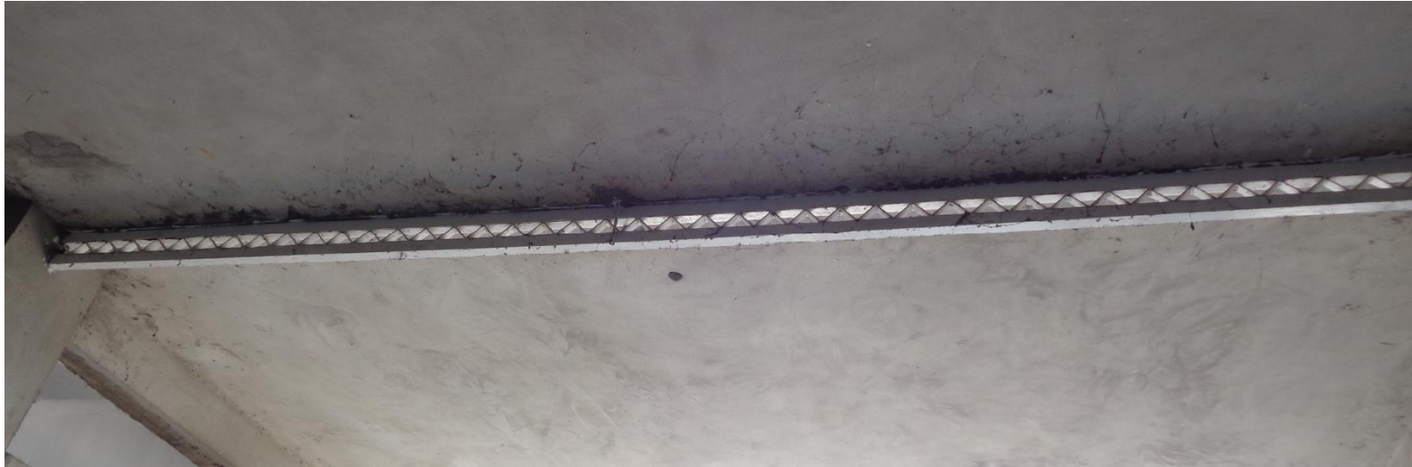
Below first floor slab of front building - entrance
