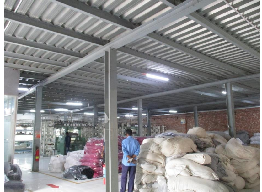
Portal frame at ground floor
