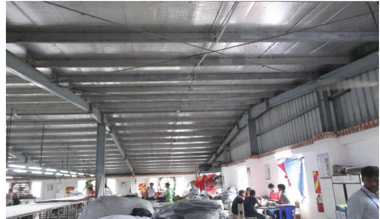
Roof system on site
