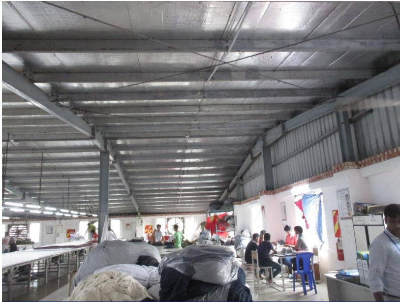
Portal frame at 1 st floor
