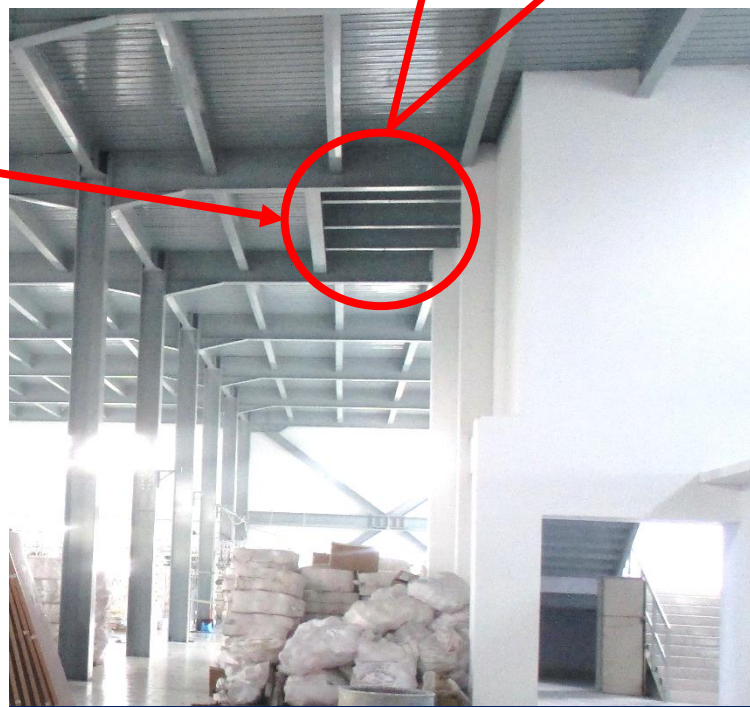
Three beams found on site
