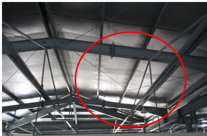
Loosely tied vertical cable bracing at east side
