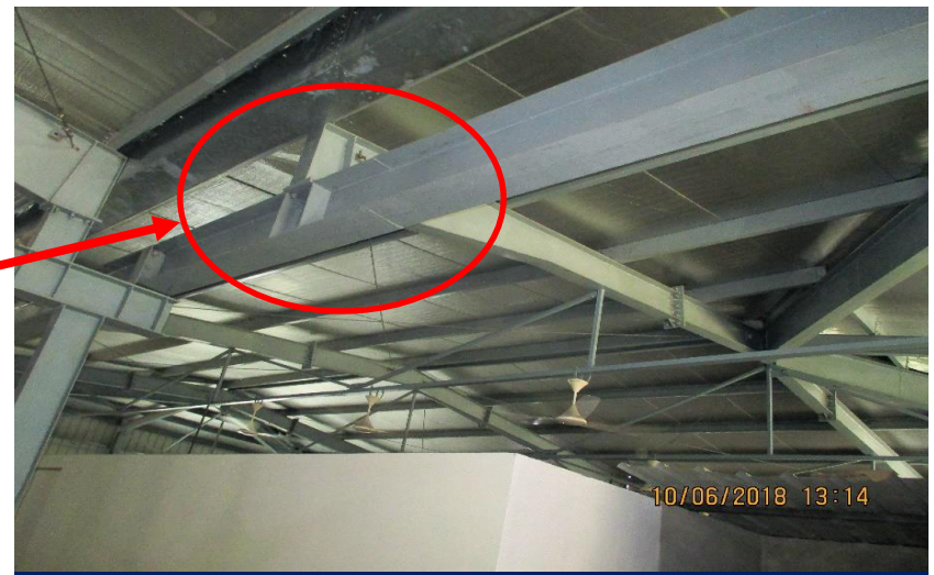
Jack beam supporting rafters
