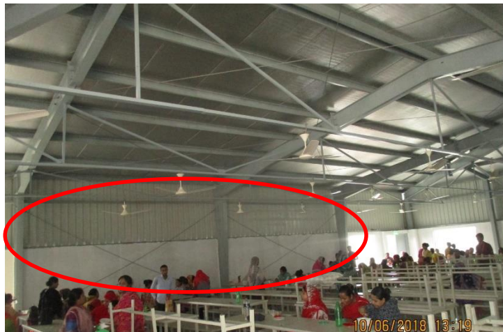
Loosely tied vertical cable bracing at east side
