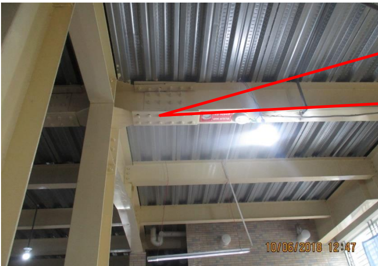
Improper connection was observed in ground floor at column and beam joint
