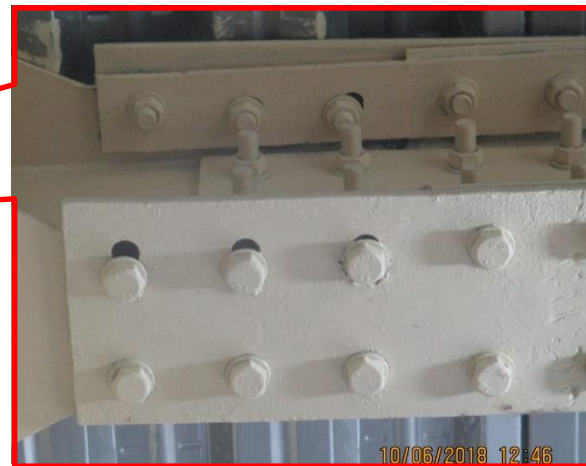
Improper connection was observed in ground floor at column and beam joint
