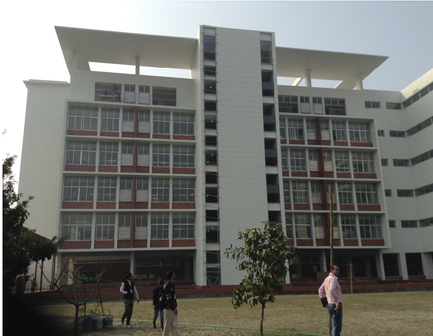
Front Elevation of Factory Building (North)
