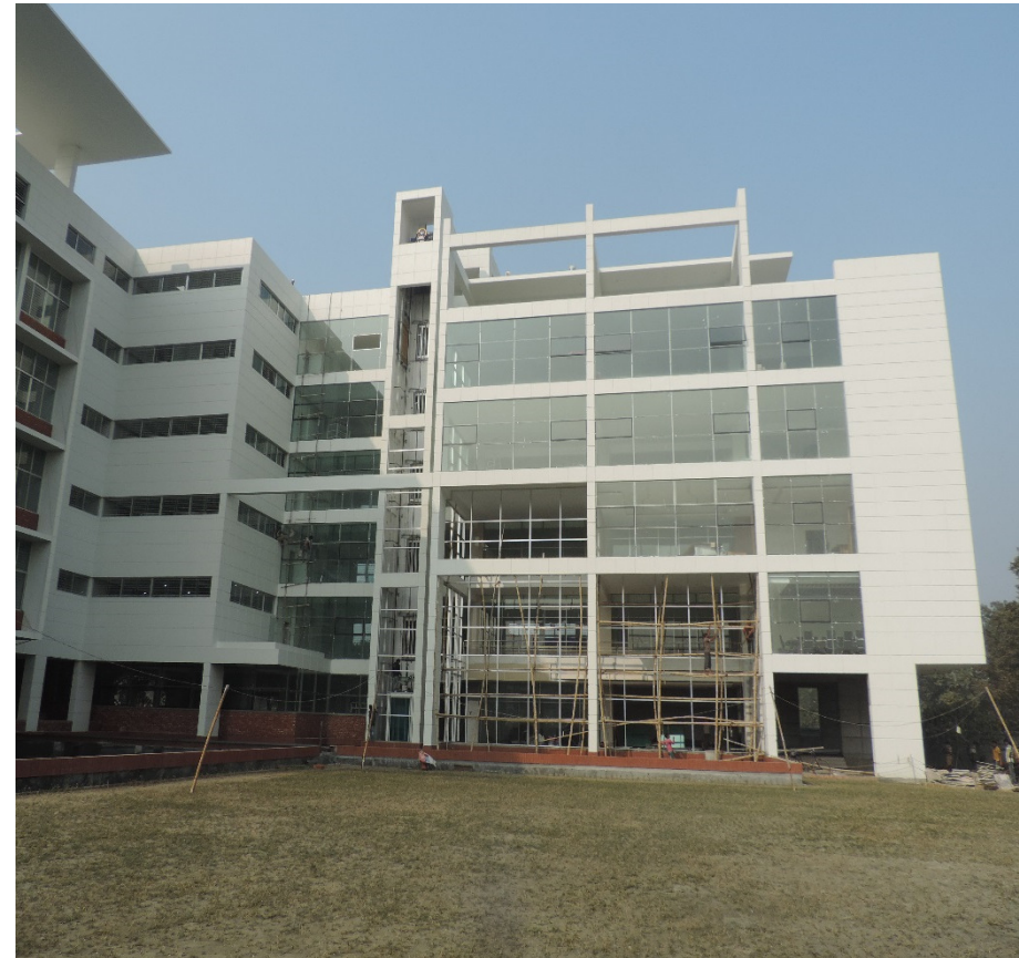
East Elevation of Office Building connected with Factory Building
