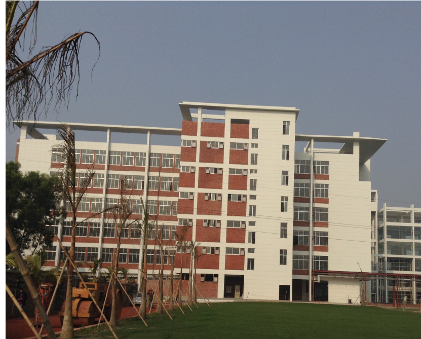
East Elevation of Factory Building
