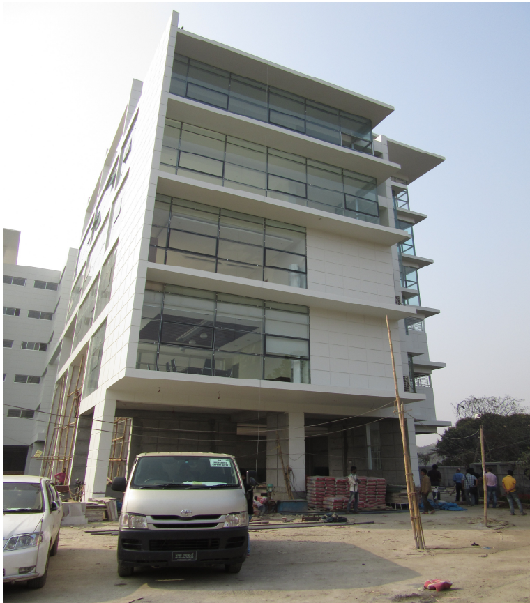
Front Elevation of Office Building (North)
