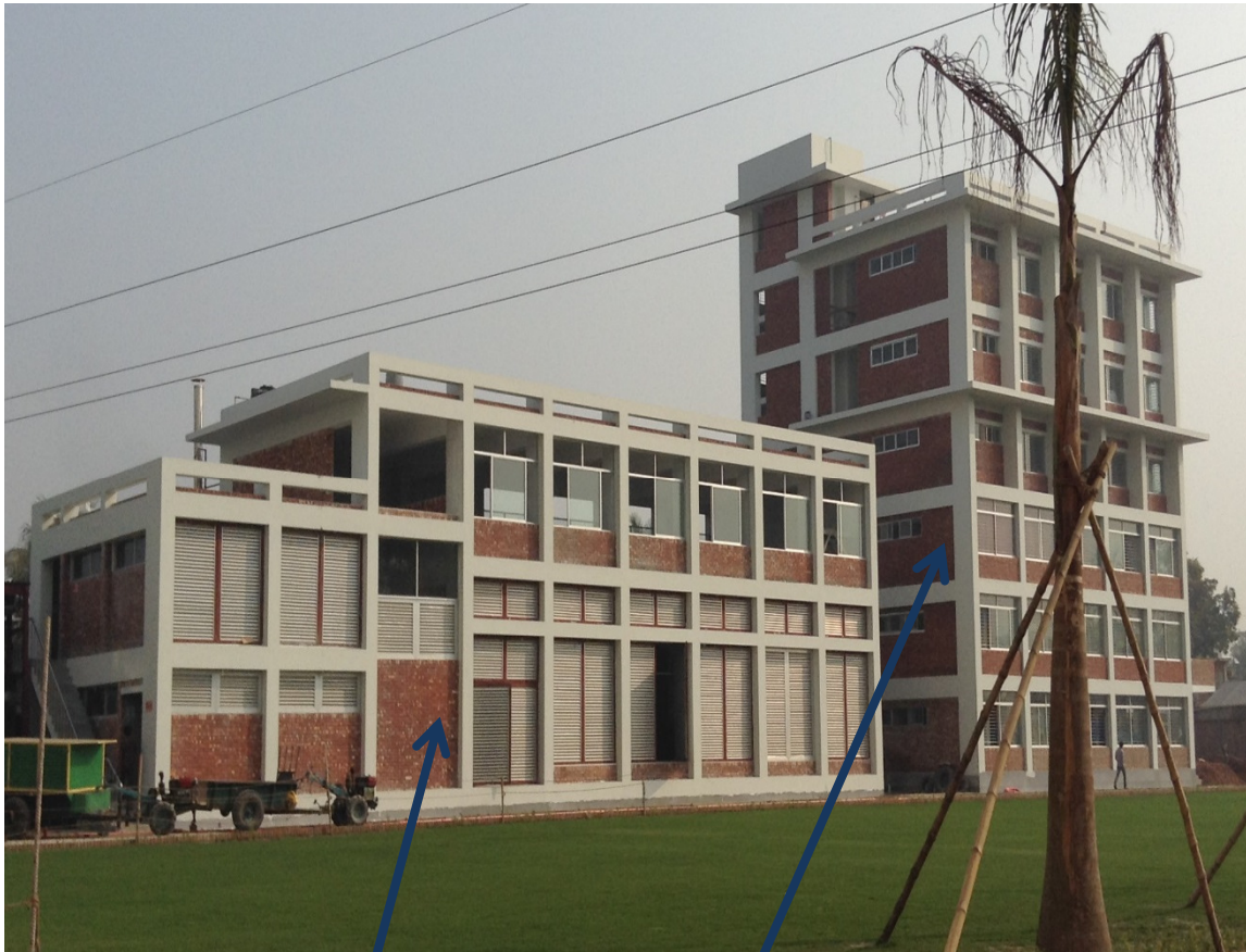
Energy Building & Security Building (South-West View)
