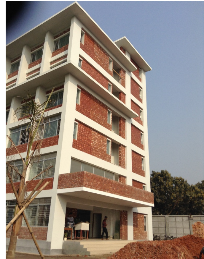
Front Elevation of Security Building (East)
