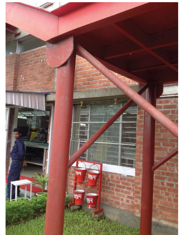
Steel stairs (east)
