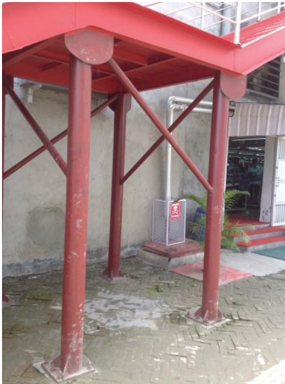
Steel stairs (west)
