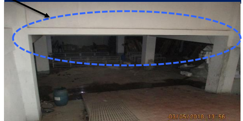
The marked beams were absent in basement floor on ramp area but the beam was shown in drawing.
