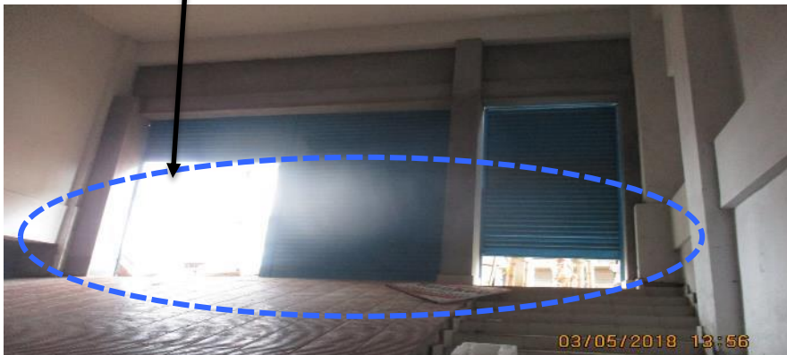
The marked beams were absent in basement floor on ramp area but the beam was shown in drawing.
