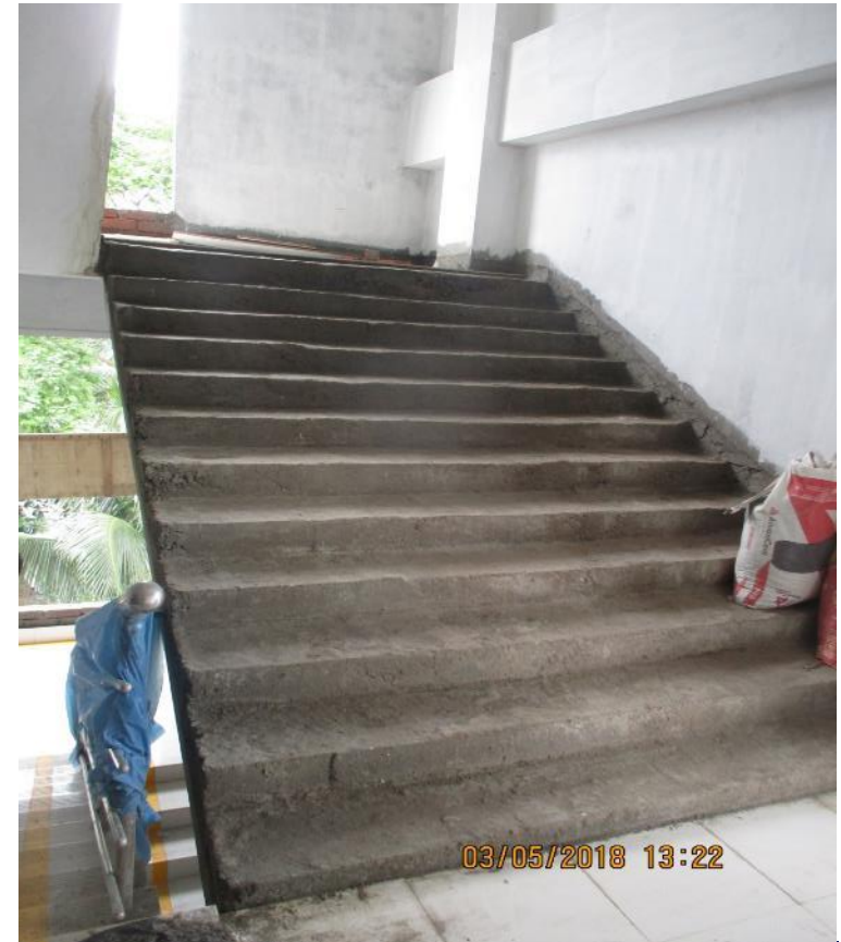
South-West stair case portion.
