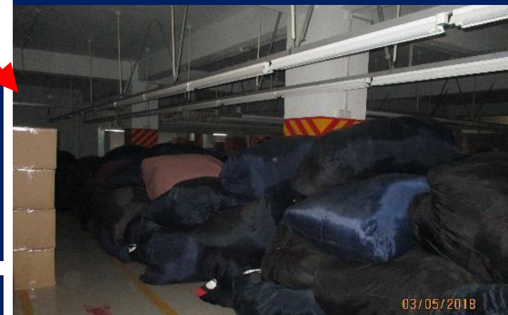
Uncontrolled loading exceeds 3 kPa
