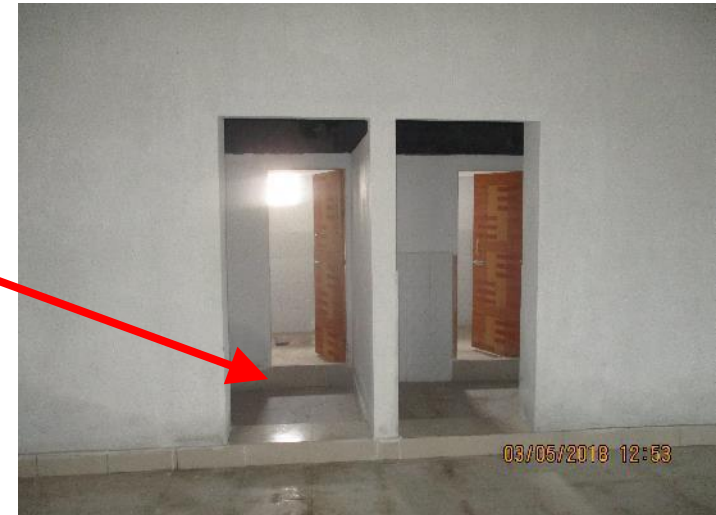
120~380 mm build up area in toilet zone.
