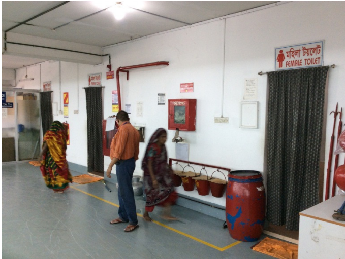
Toilet Build-up + partition walls
