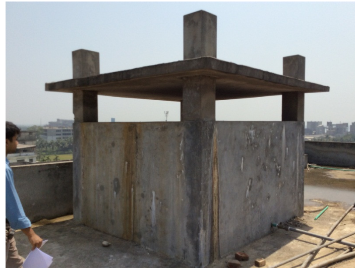
Water tank on top of lift shaft
