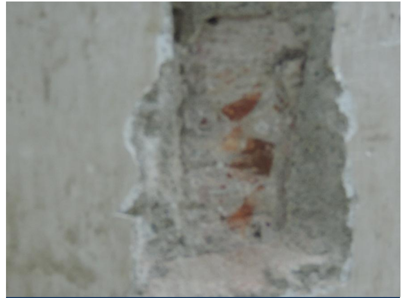
Brick aggregate in column
