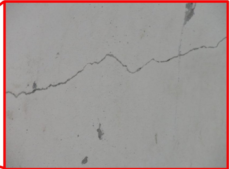
Crack in wall panel
