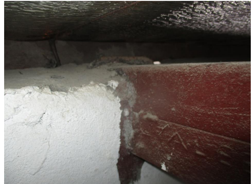
Rafter connection with brick wall
