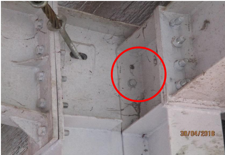
Missing Bolt at several locations
