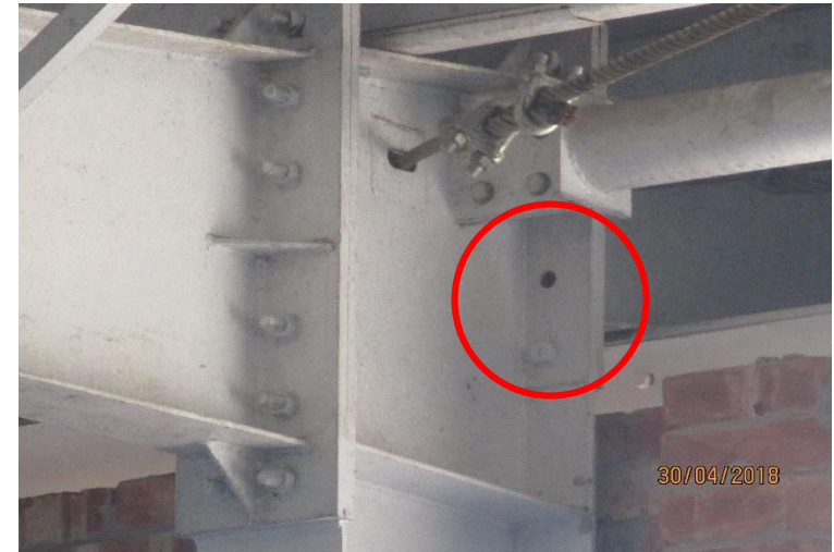
Missing Bolt at several locations
