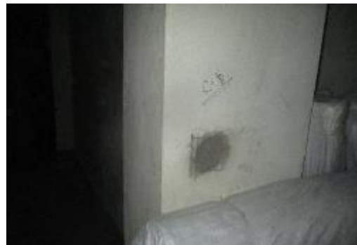
Core cutting location
