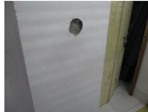
Core cutting location
