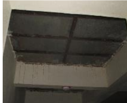
Steel sheet poorly connected with RC slab by welding
