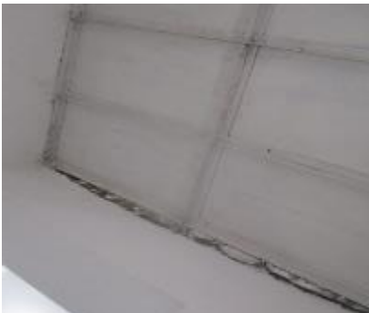
Steel sheet poorly connected with RC slab by welding
