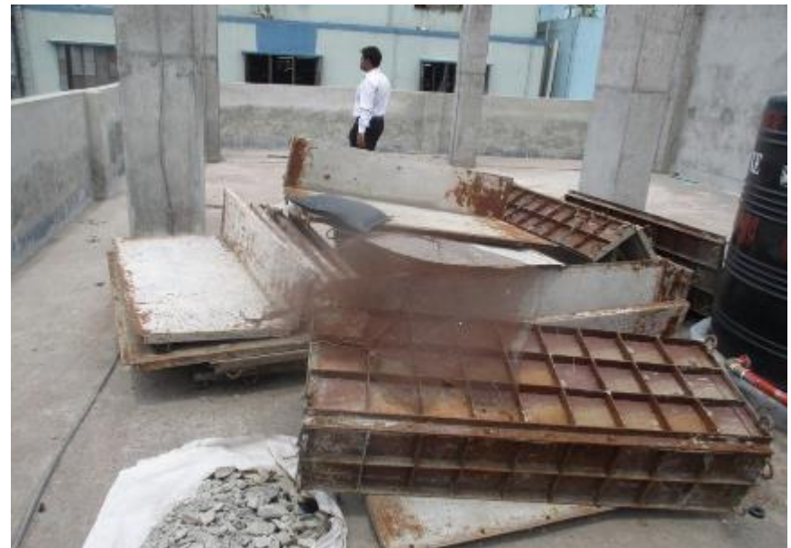
Stacking of construction materials
