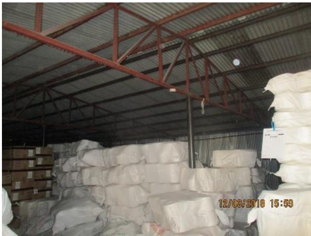
Typical truss frame with out any horizontal or vertical bracing system in Grey fabric store
