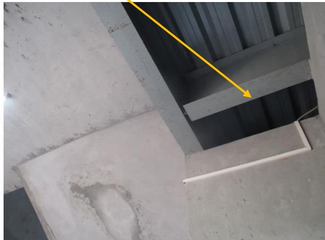
Sub-Beam near stair
