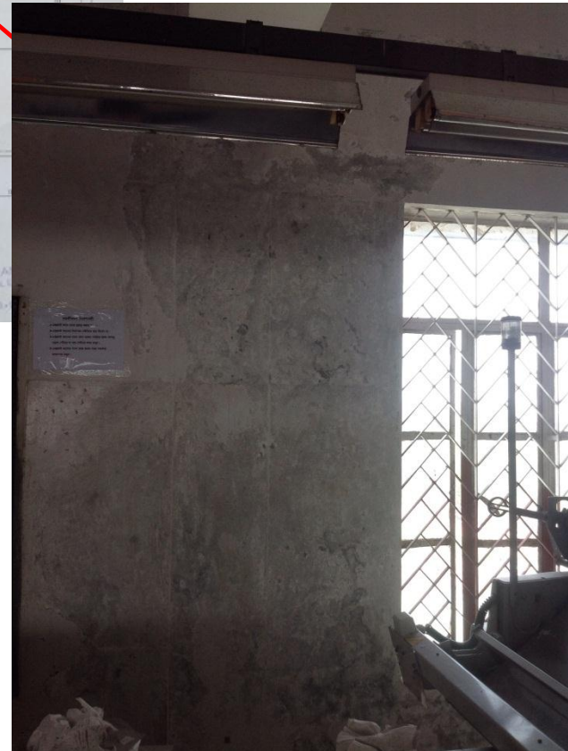
Water ingress on 4 th floor of 6 storey building
