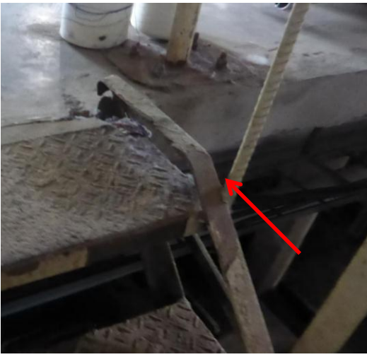
Stairs have limited independent lateral stability systems and poor connections to neighbouring buildings.
