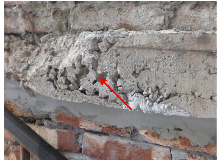
Poor compaction of concrete in columns and other structural elements observed.
