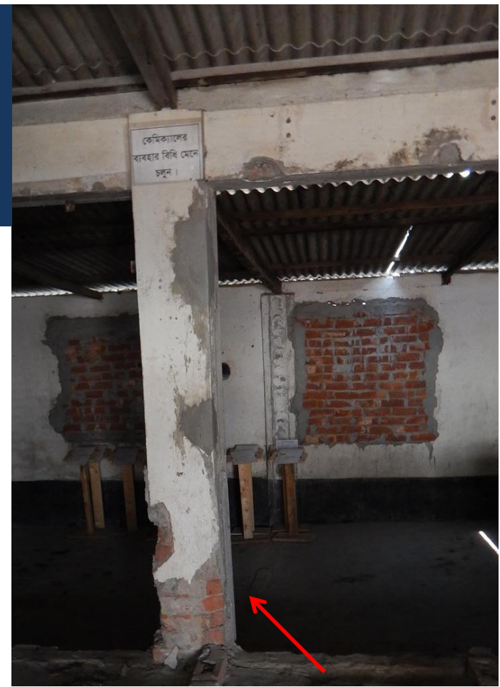
Masonry piers used to support concrete beams.
