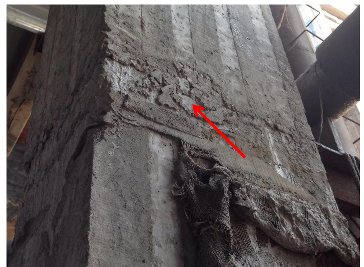
Poor compaction of concrete in columns and other structural elements observed.
