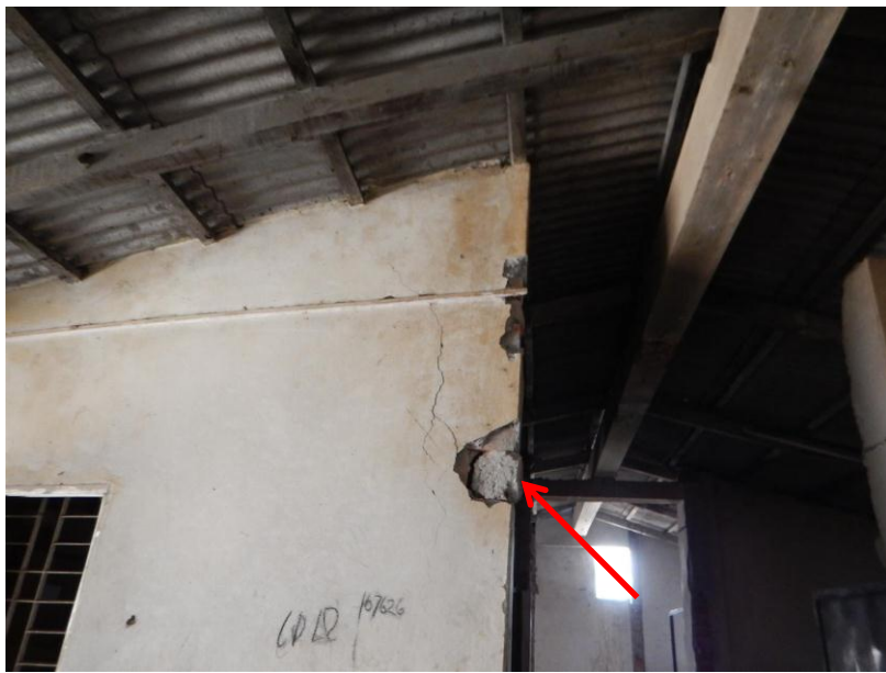
Masonry piers used to support concrete beams.
