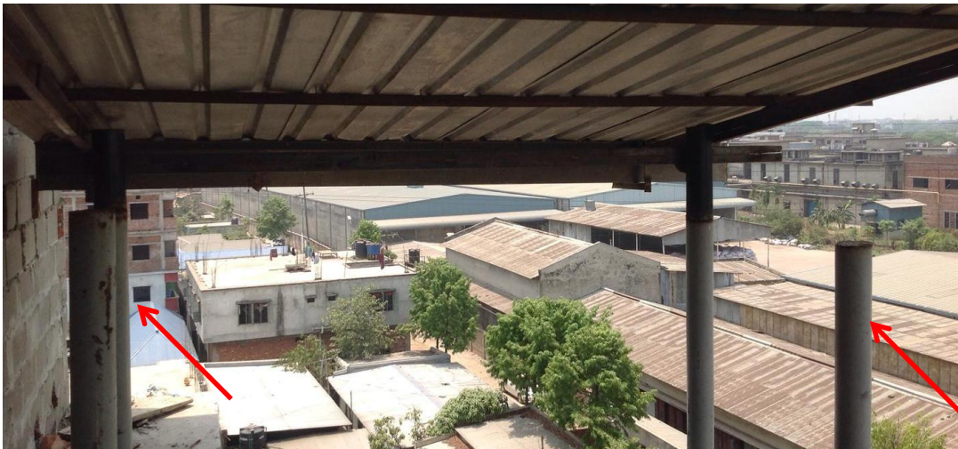
Stairs have limited independent lateral stability systems and poor connections to neighbouring buildings.
