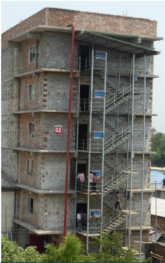
Escape stairs to Building 2
