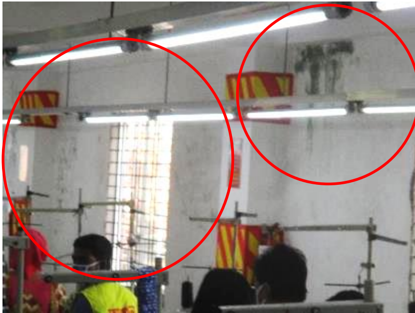
Dampness on periphery wall of 5-storied portion
