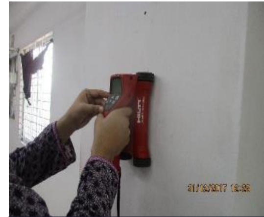
Rebar checking with Ferro scanning of Column
