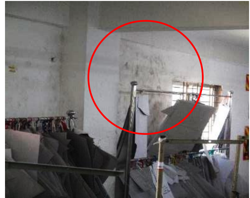
Dampness on periphery wall of 5-storied portion
