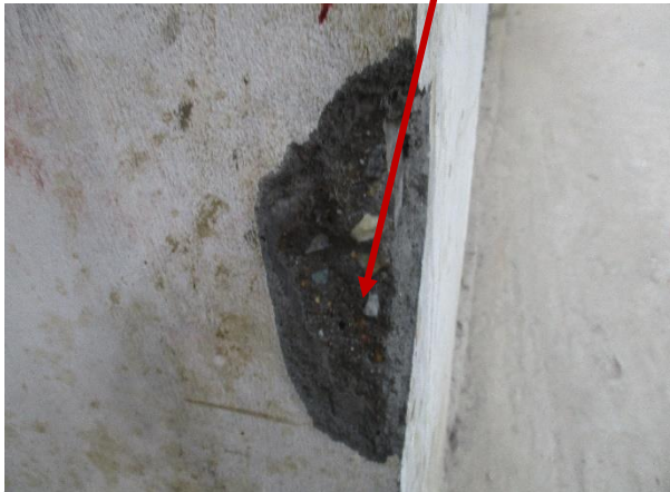
Stone chips aggregate at strengthened column
