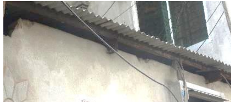
Lightweight steel roof rested on the brick walls
