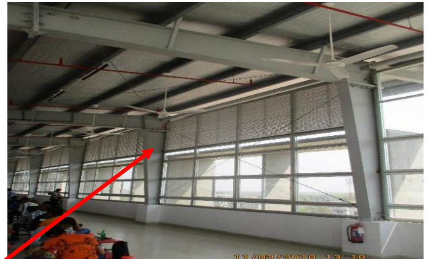
In place of SB1 beam, pipe Compression Strut was installed
