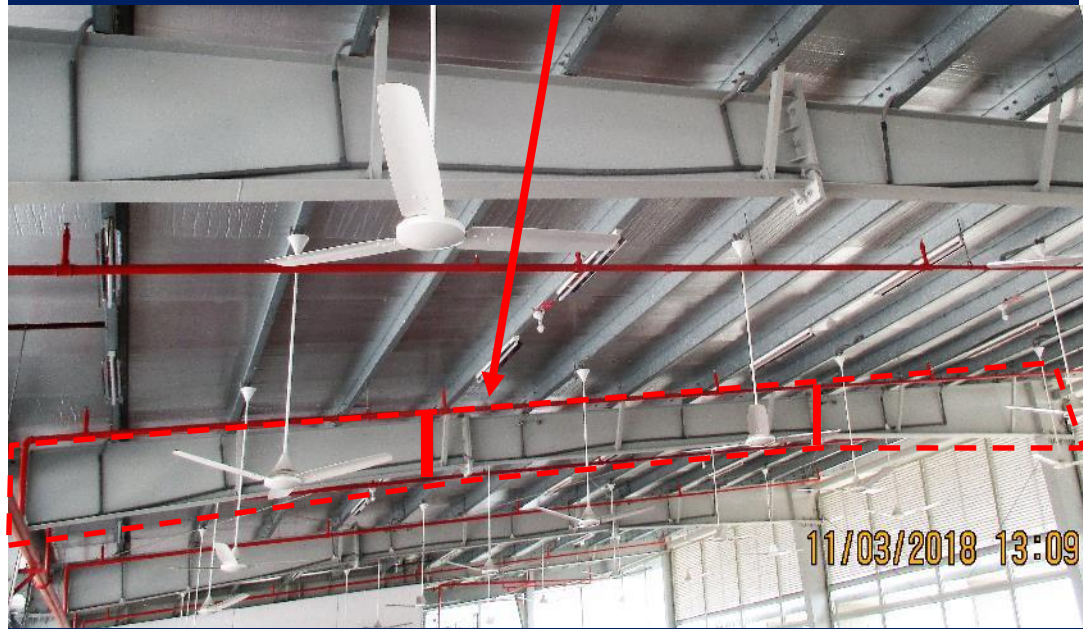
Internal view of roof top shed
