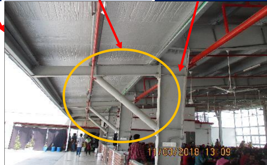
Columns in north side with knee bracing
