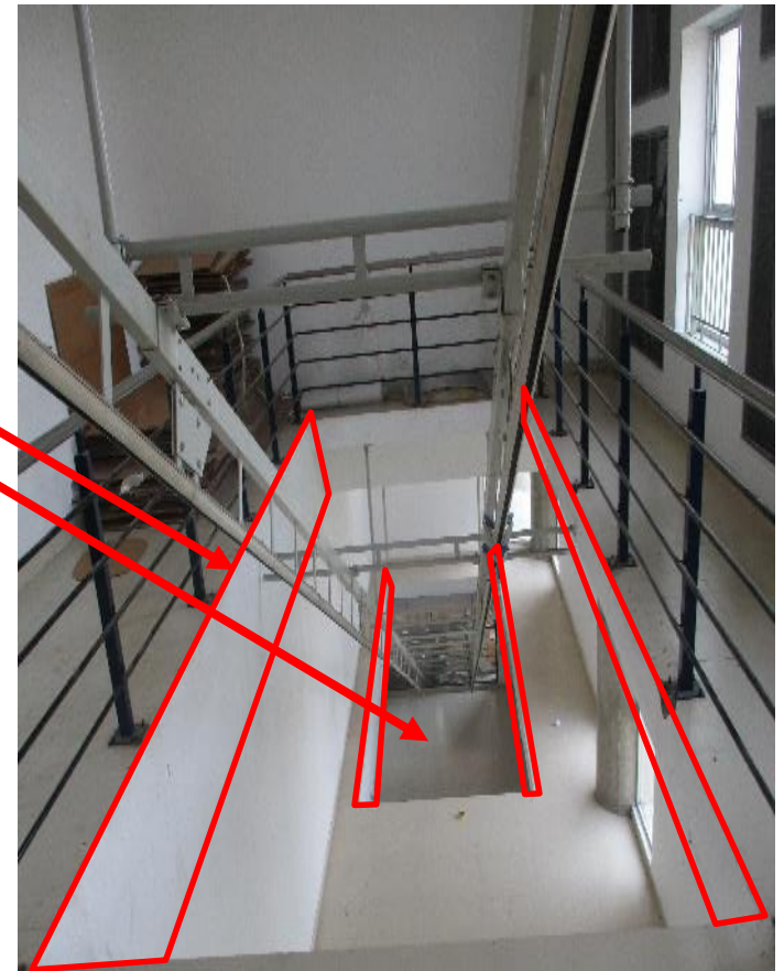
Opening in slab due to conveyor facilities
