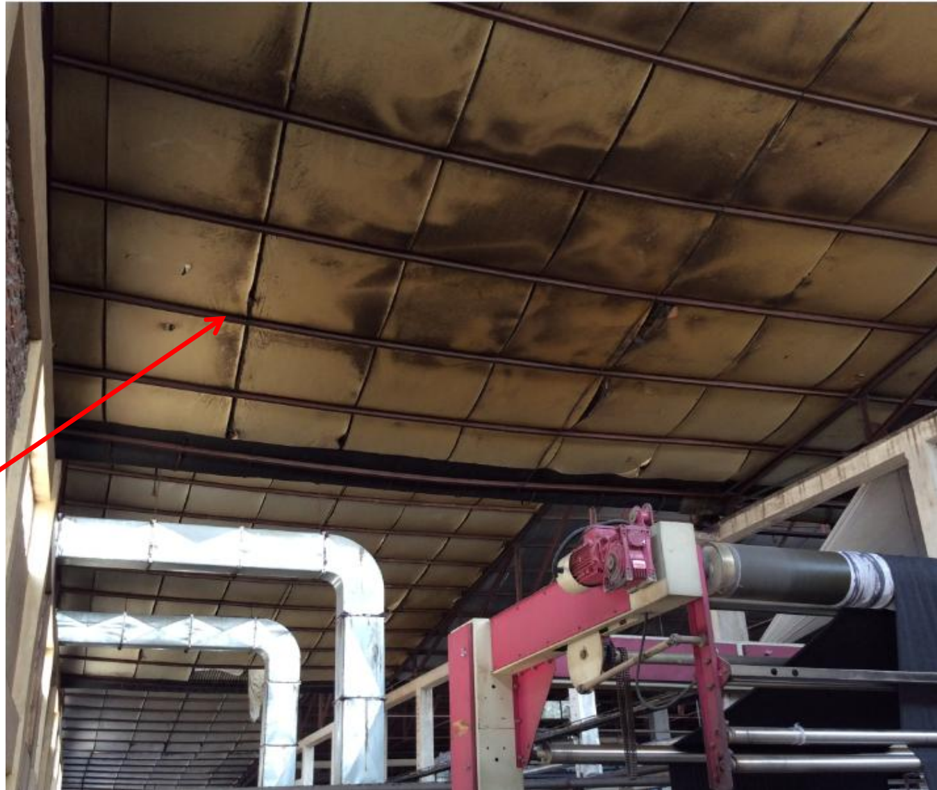
Single-Storey Building: Dyeing Shed
