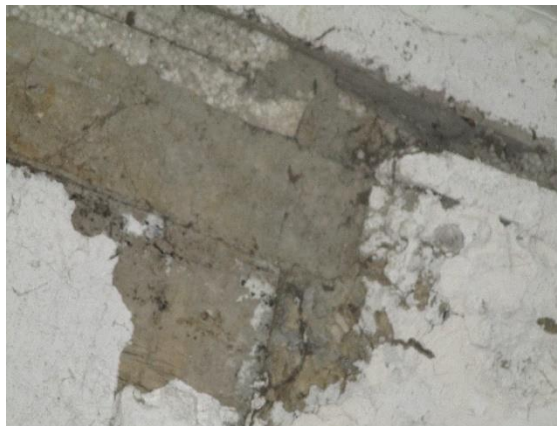
Loose filler material through isolation gap
