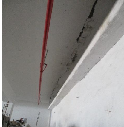
Loose filler material through isolation gap
