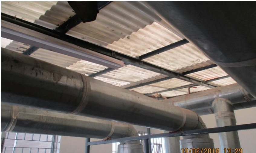
Internal roof frame
