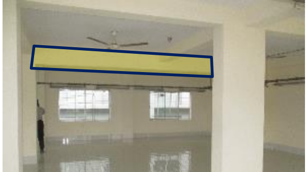
Down Stand of the highlighted (yellow marked) beam was observed 450 mm instead of 325 mm on GF and 1st Floor
