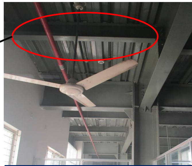
Detail of SB-3 type sub-beam was absent in drawing
