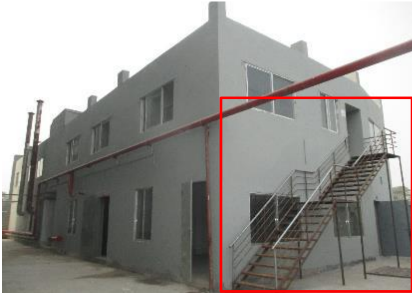
Steel Stair outside of the utility building
