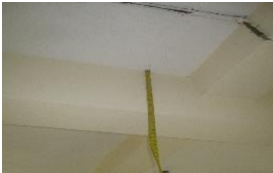
Down Stand of the highlighted (yellow marked) beam was observed 450 mm instead of 325 mm on GF and 1st Floor
