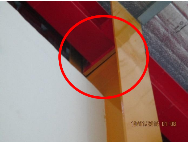
Existence of significant gap at connection
