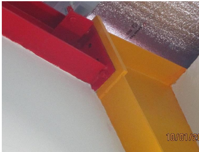
Bolts missing in several location
