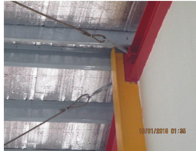
Bolts missing in several location
