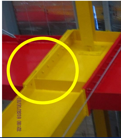
Bolts missing in several location
