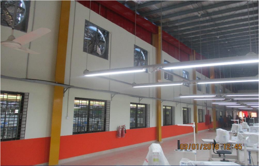
No vertical bracing on site
