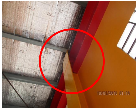
Existence of significant gap at connection
