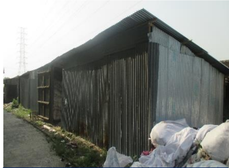
Non engineered shed in Wastage Store
