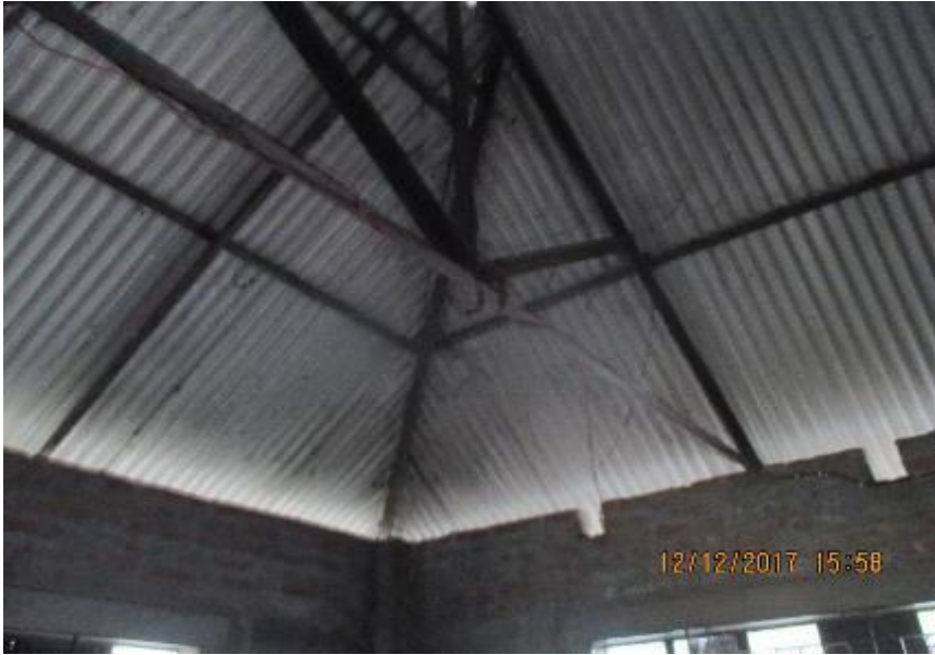
Truss Shed resting on the brick wall in staff canteen
