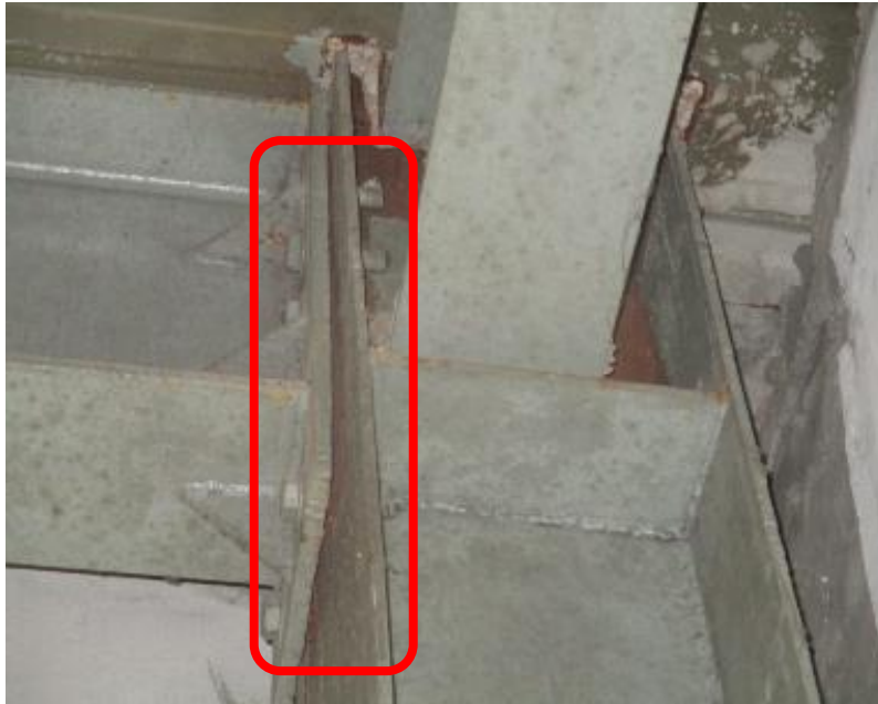
Gap in between beam-column joint
