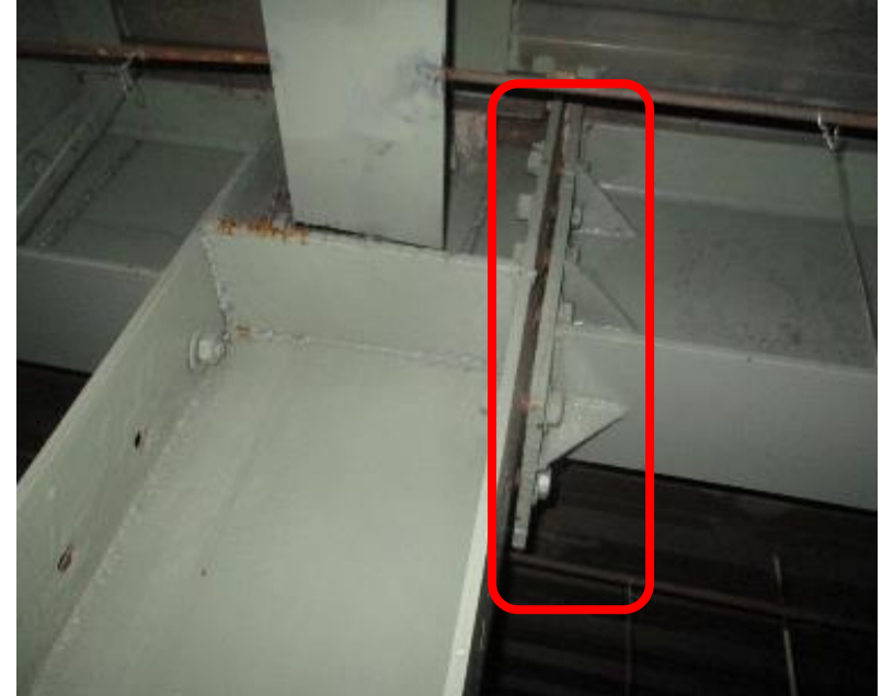
Gap in between beam-column joint
