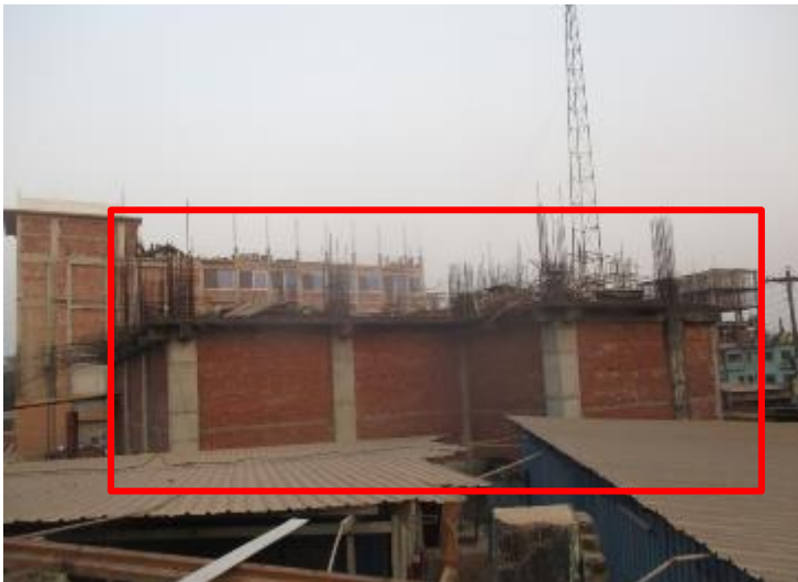
Current condition of the building
