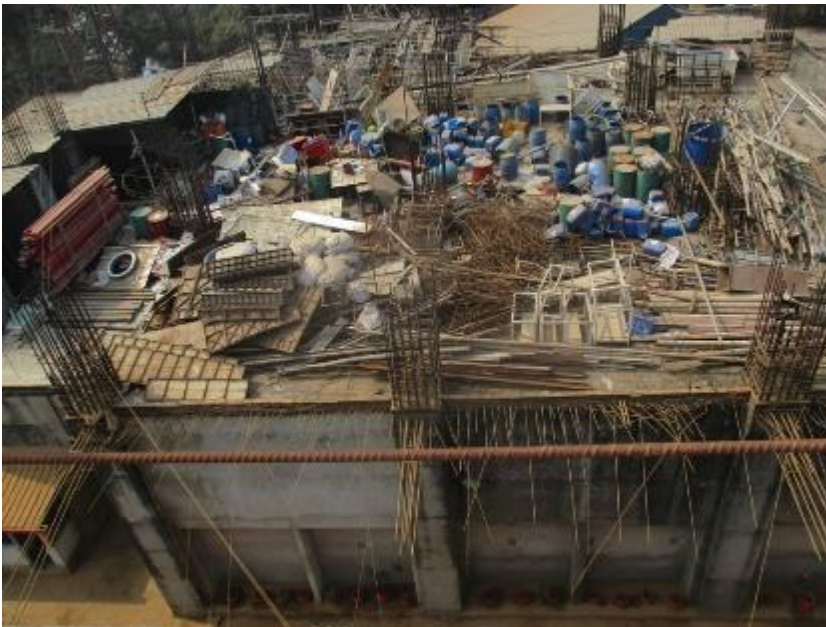
Ground floor roof.
