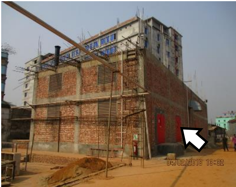
Current condition of utility building
