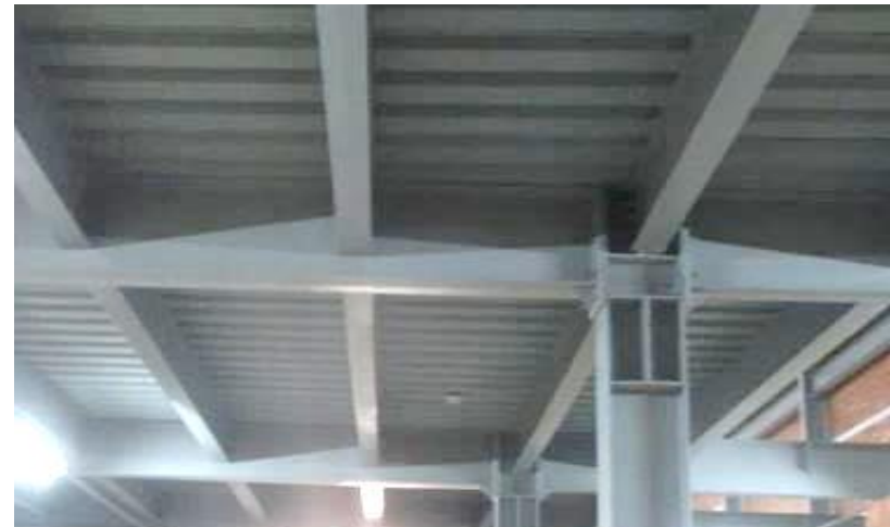
Typical beam-column connection
