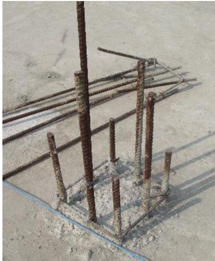
Exposed reinforcements on the roof
