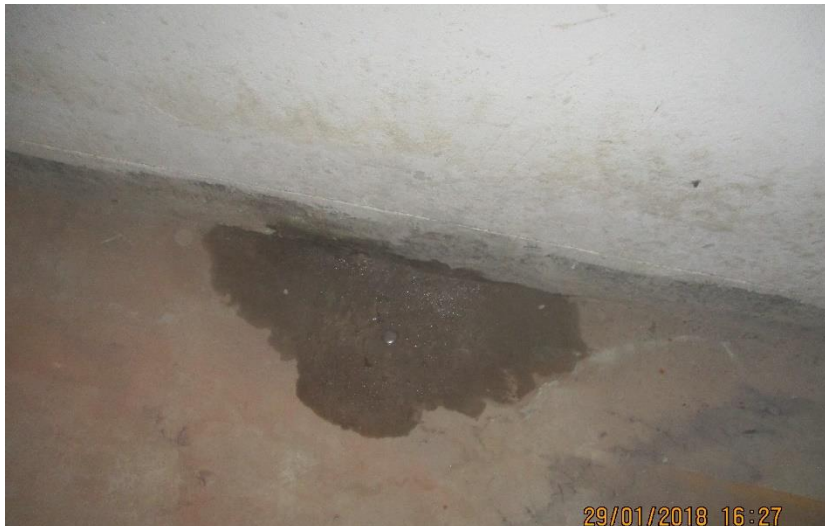
Water seeping and formation of minor cracks
