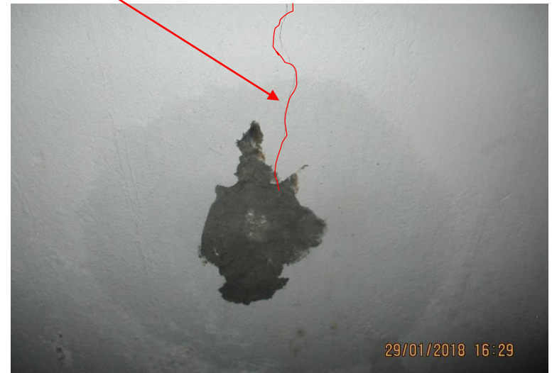
Water seeping and formation of minor cracks
