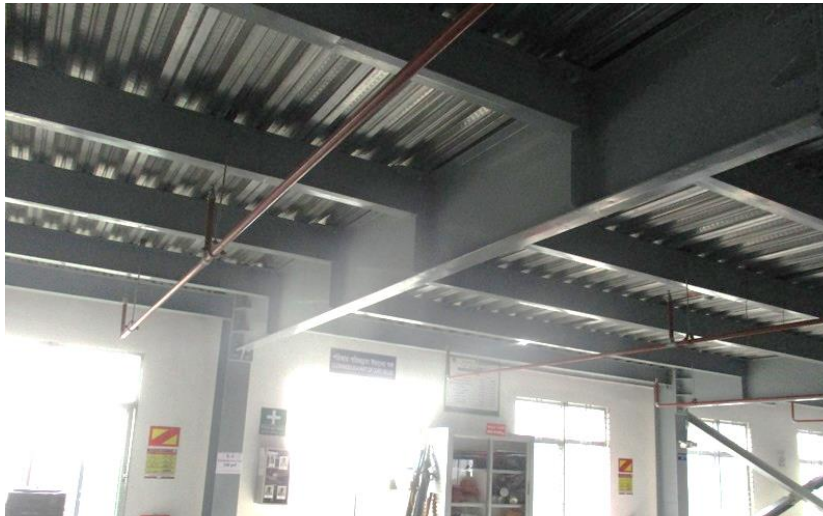
Sub-beam at 5 th floor
