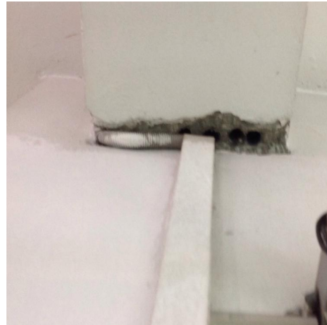
Soffit of 2 nd Floor
