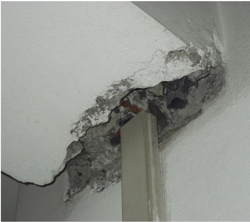
Soffit of 3 rd Floor
