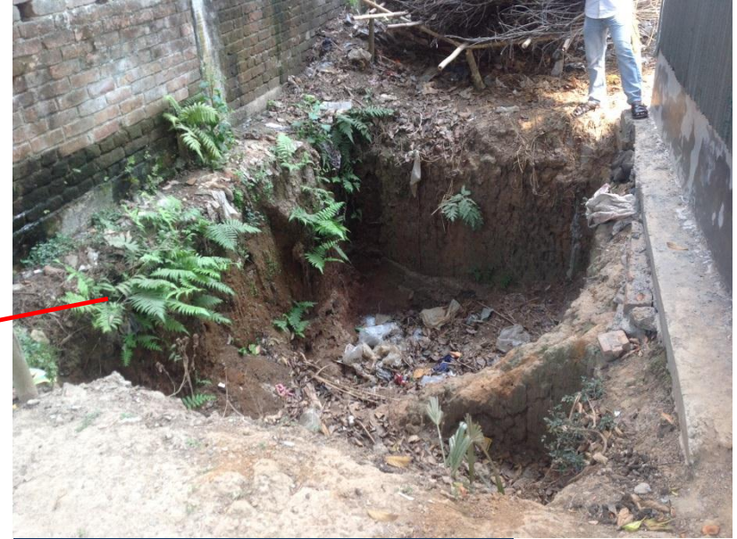
Excavation at building perimeter
