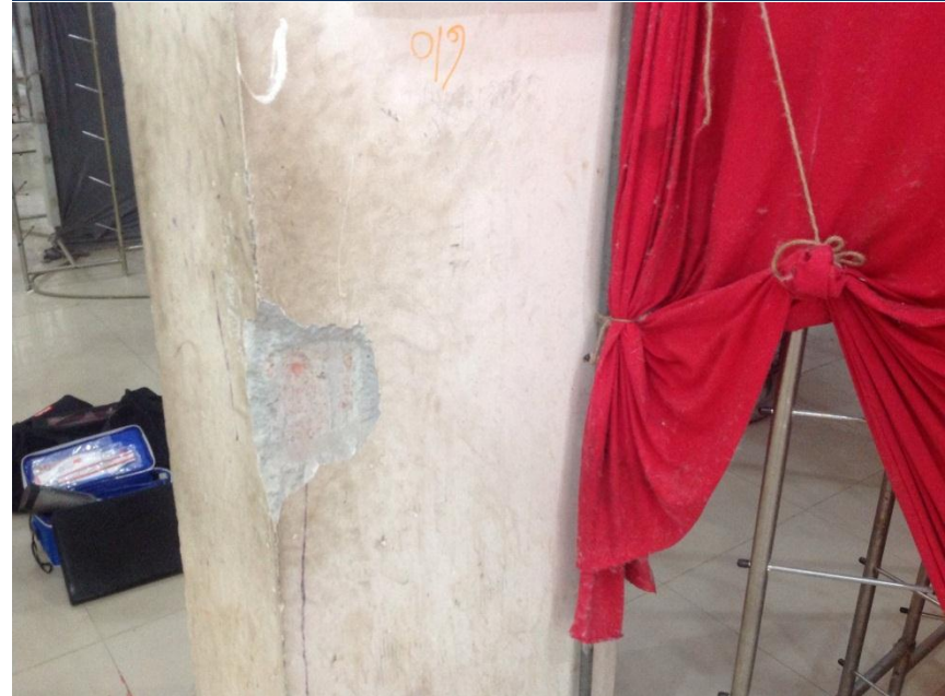
Ground Floor Column
