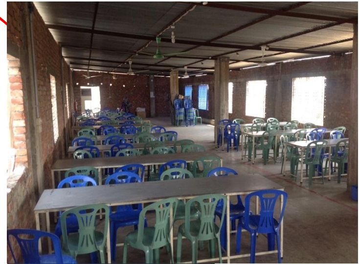
Additional roof structure
