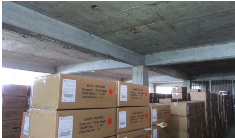
Beam and slab of existing site
