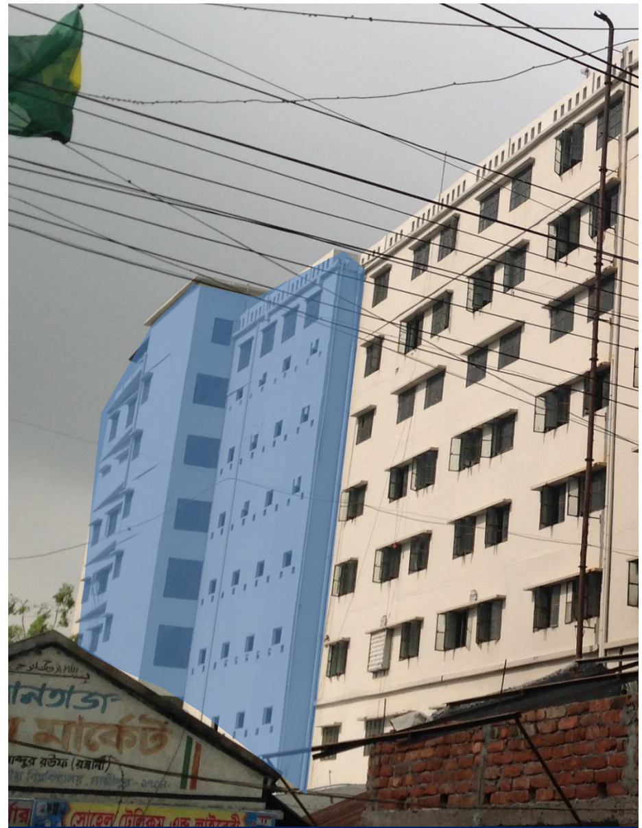
Cantilever structure to the Southwest of the N-S Building
