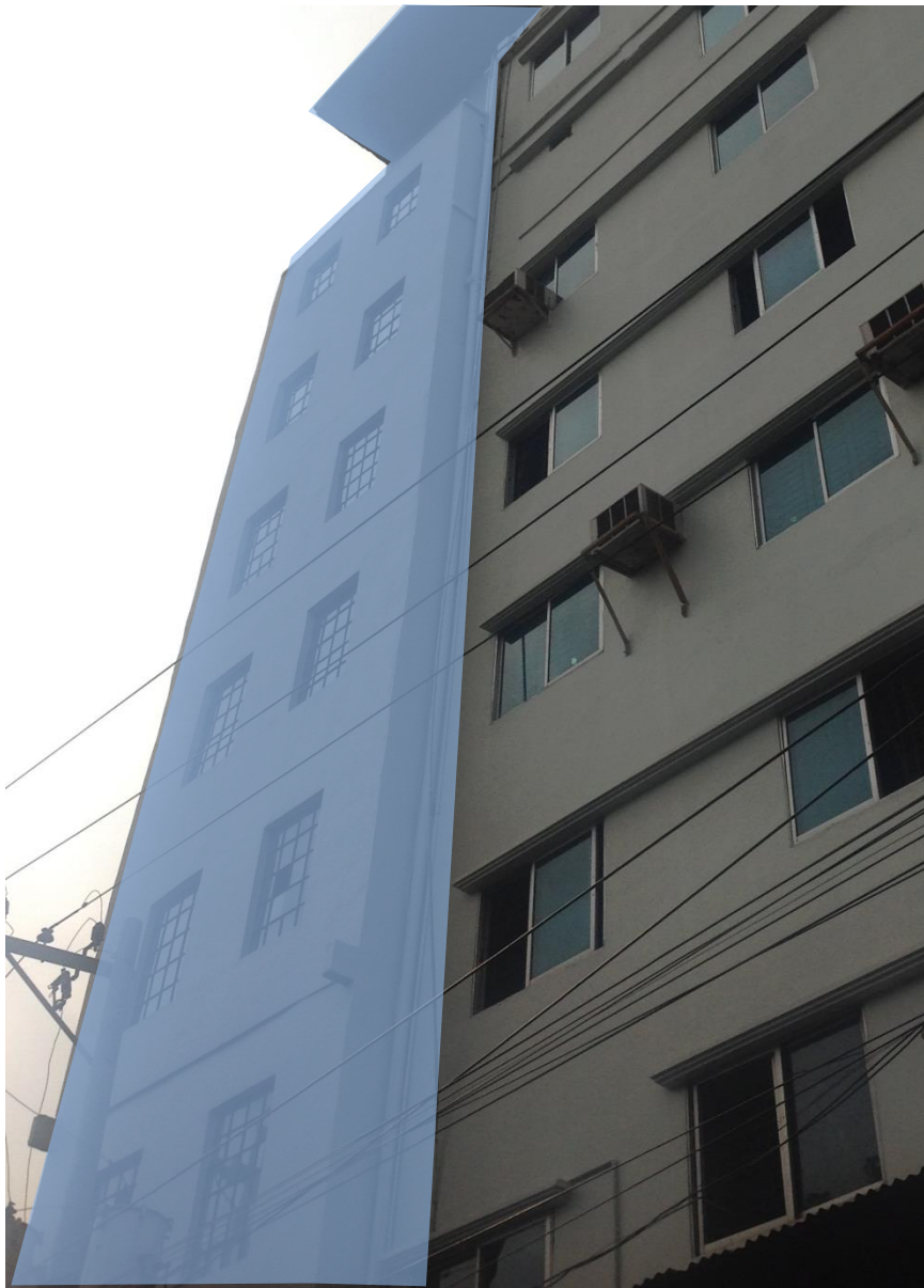
Cantilever structure to North of N-S Building
