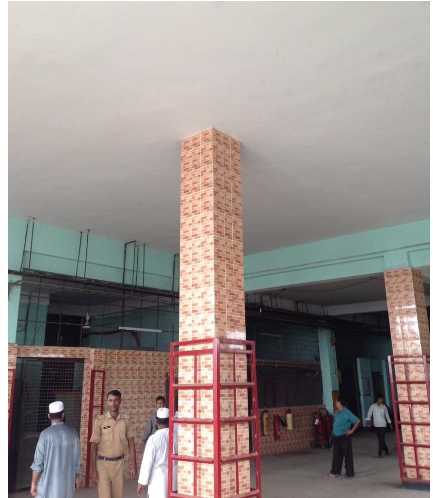
Angle steel frames at columns
