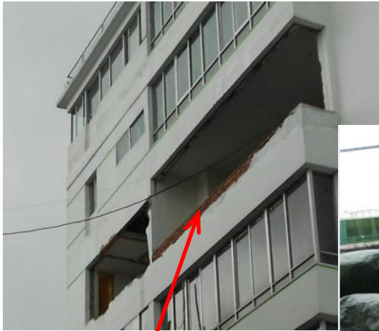
Ongoing works (new bathrooms)
