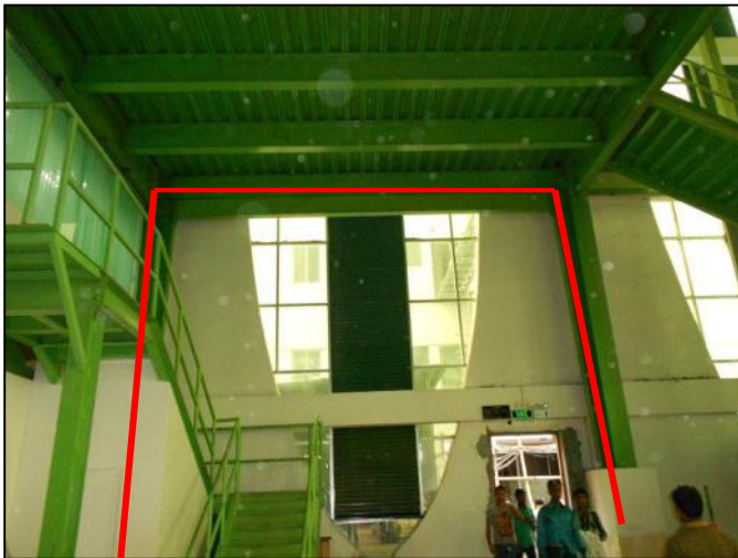
Additional moment frames (MF) – purpose and capacity unknown
