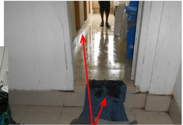
250 – 350mm new build-up at new bathroom.
