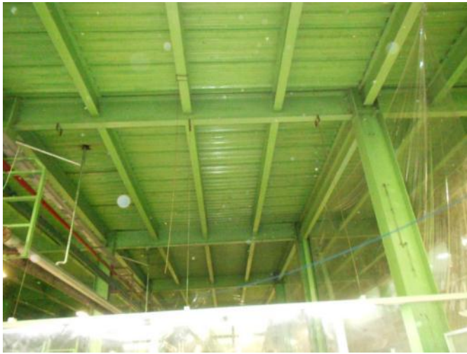
General floor beam arrangement
