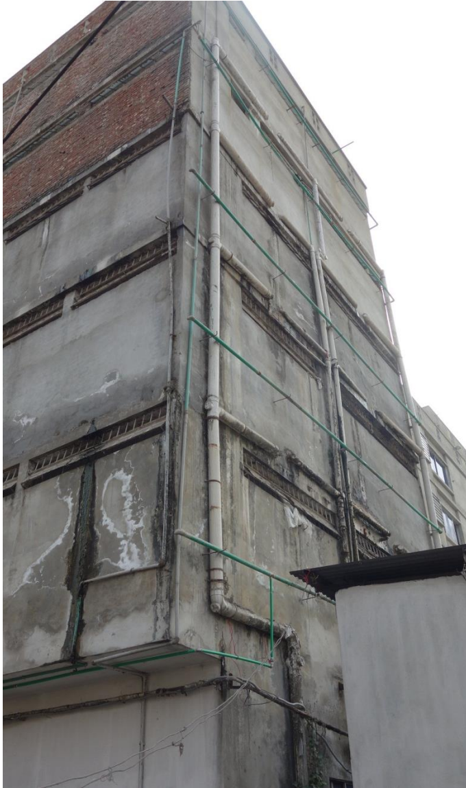
Leaking drainage pipes on façade. Running water visible.
