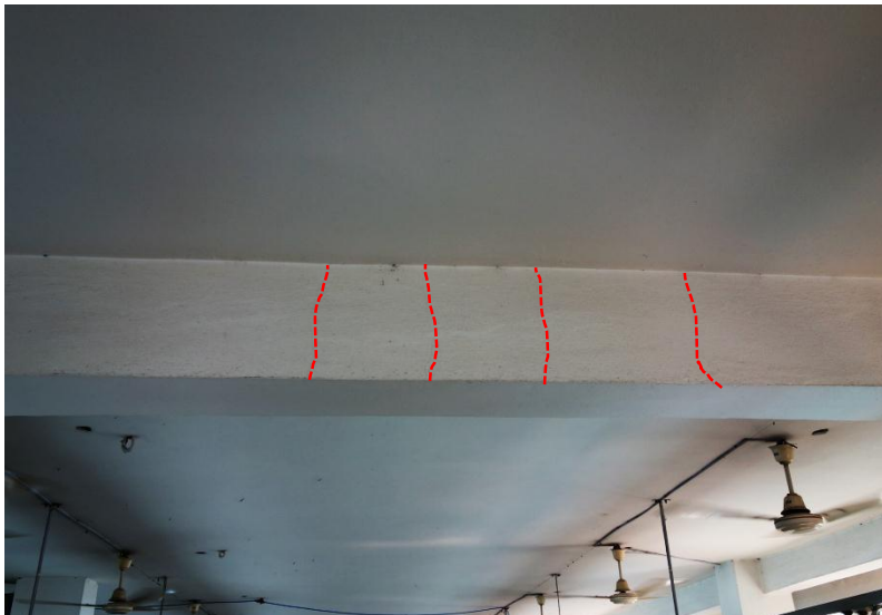
Cracking in beams at level 3
