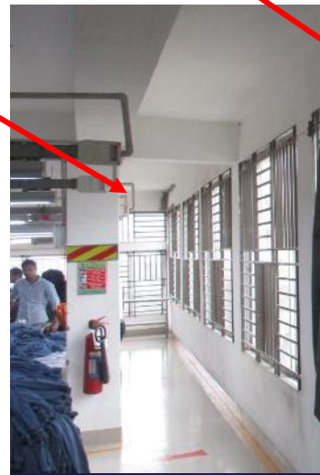
Both uniformed and tapered beams were found on south side however the beams were not mentioned in drawing
