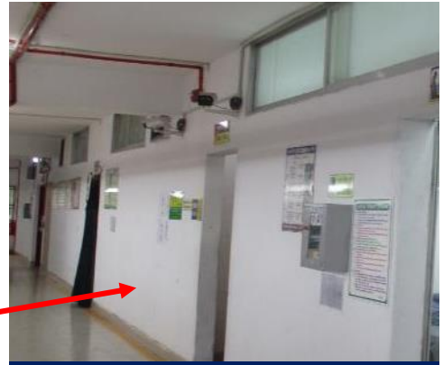
125mm built-up and 125mm thick outer brick wall on toilet area
