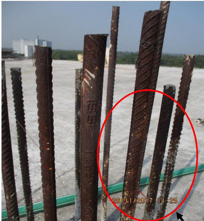
Exposed Rebar on roof top tends to corrosion
