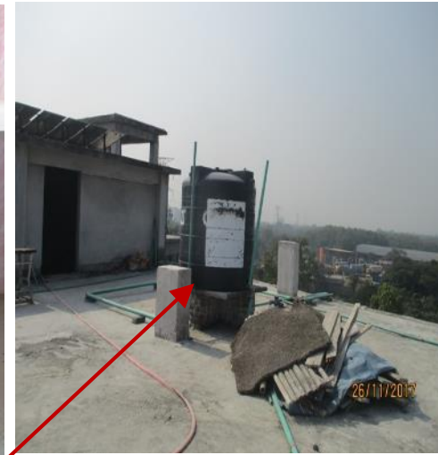
Water reservoir at roof
