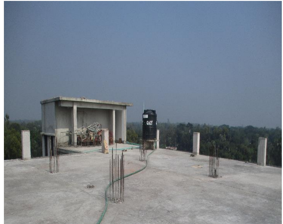
Exposed Rebar on roof top tends to corrosion
