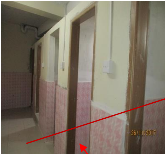
Toilet Zone with masonry walls
