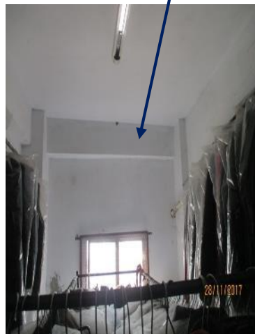
Beam Size measured 300mm (w) x 350mm (d/s)
