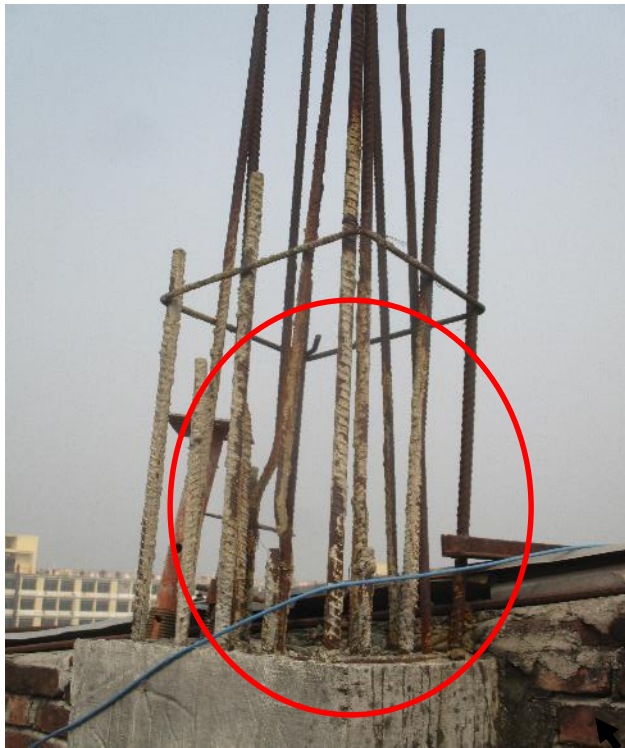
Exposed Rebar on roof top tends to corrosion
