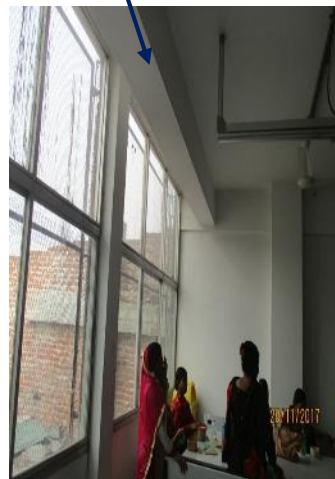
Beam Size measured 300mm (w) x 350mm (d/s)
