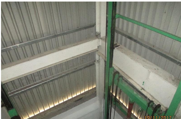
Additional columns for cargo lift and toilet zone were not shown in column layout. Also thickness of flange was measured 6mm but in column section it shows 8mm.
