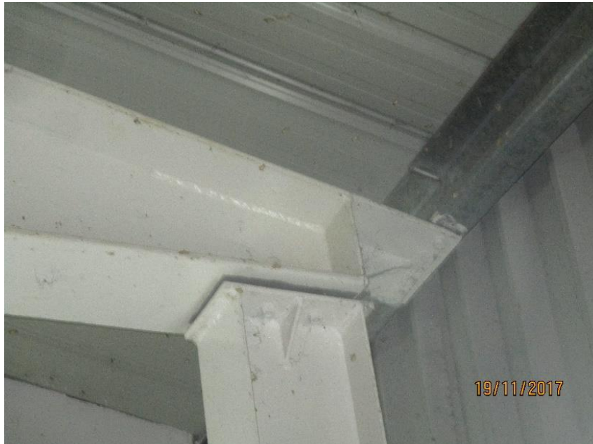
Gap found in between column and rafter at toilet zone
