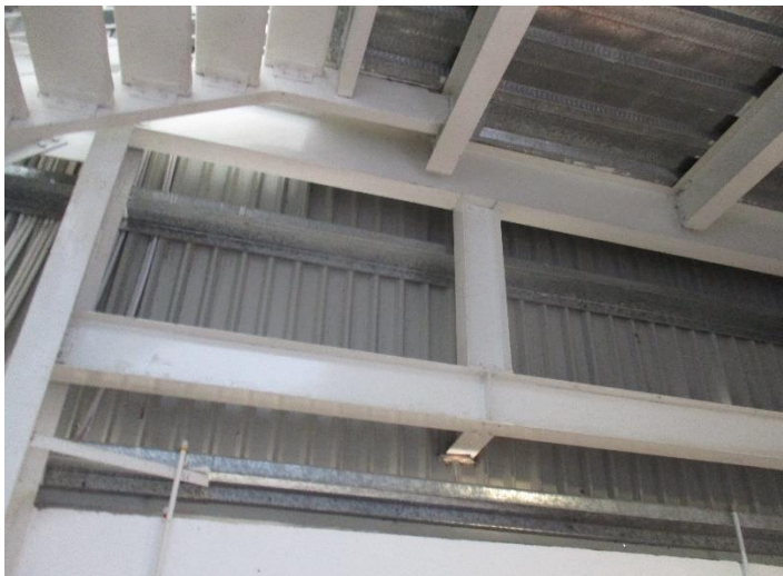
Additional short column in gable frame was not shown in drawing
