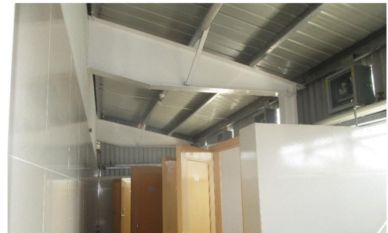
Additional columns for cargo lift and toilet zone were not shown in column layout. Also thickness of flange was measured 6mm but in column section it shows 8mm.
