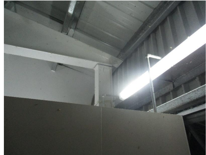
Gap found in between column and rafter at toilet zone
