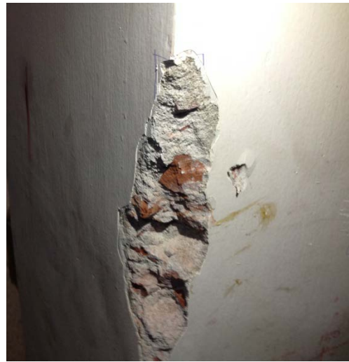
Tested column at lower floors - Brick aggregate observed.
