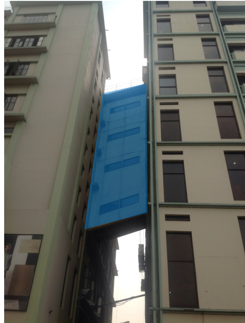
4 Storey Link Bridge between B1 and B2
