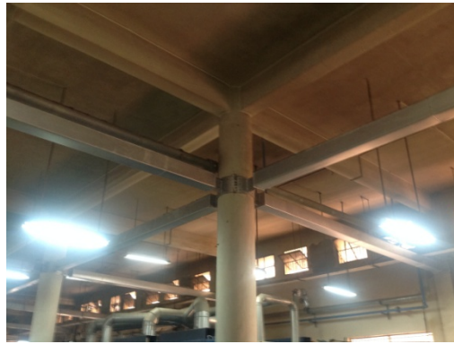
Additional steel frame for new ceiling/thermal barrier supported from structural column.
