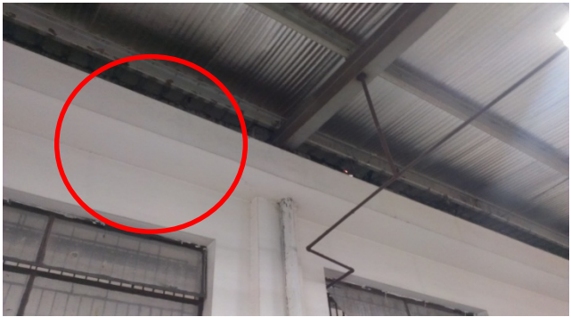
Shed extension (Building 3) supported off main building.
