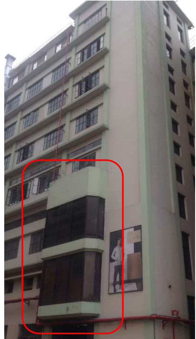
Undocumented cantilever structures from Building 2.
