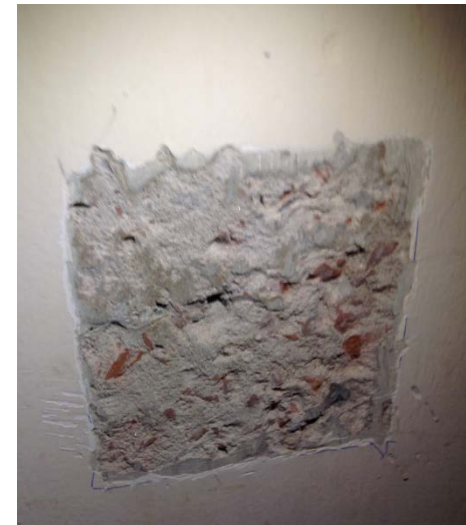
Tested column at lower floors - Brick aggregate observed.
