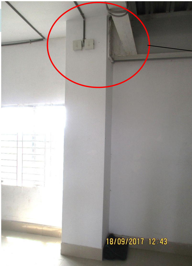
Joint between stair column (RCC) and steel beam
