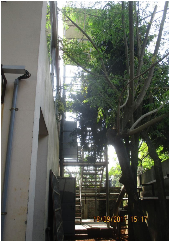
North side steel stair
