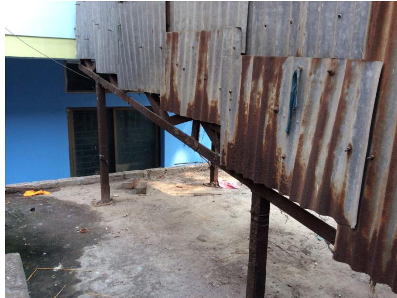
Building 2: Bridge structure deterioration
